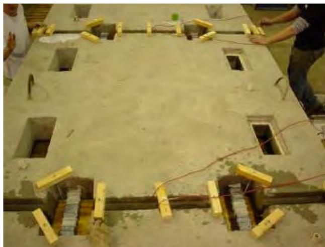
**Figure 30. Coupling Post-Tensioning Duct Across Connection**
