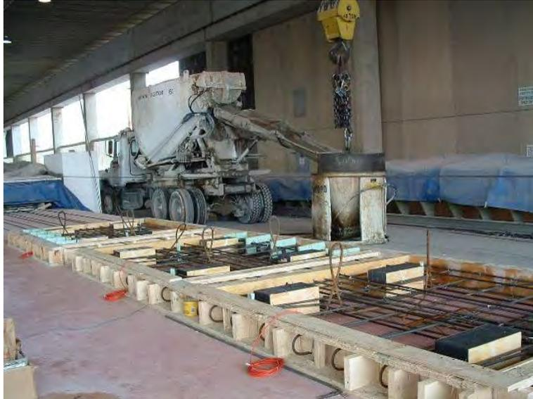
**Figure 1. Constructing Precast Panels at a Precast Plant**
