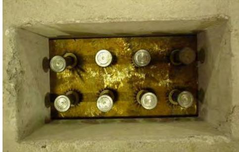
**Figure 33. Layout of Shear Studs in a Pocket**
