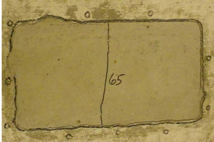
**Figure 66. Typical Shrinkage Crack Patterns in the Shear Pockets Prior to Loading**
