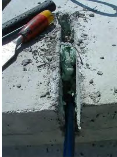
**Figure 29. Removing the EPS From the HSS Anchorage Assemblies**
