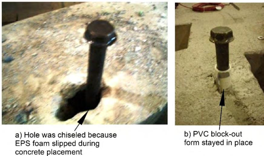
**Figure 28. Block-outs Around the Leveling Bolt Assemblies**
