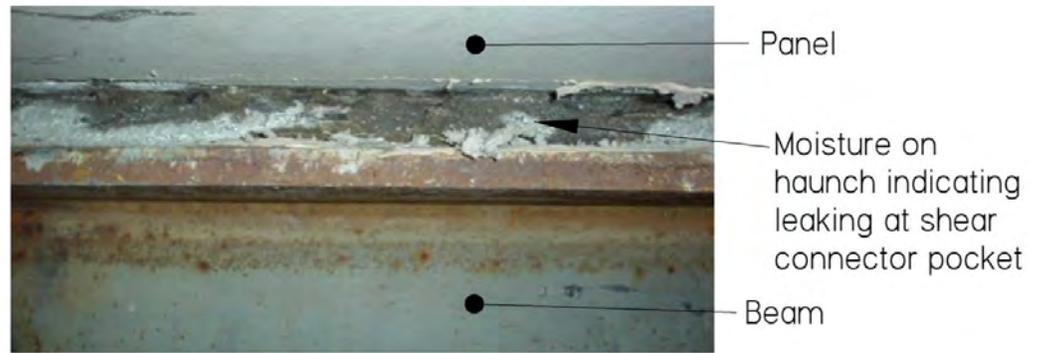
**Figure 67. Complete Leaking in the Haunch Beneath a Shear Pocket**
