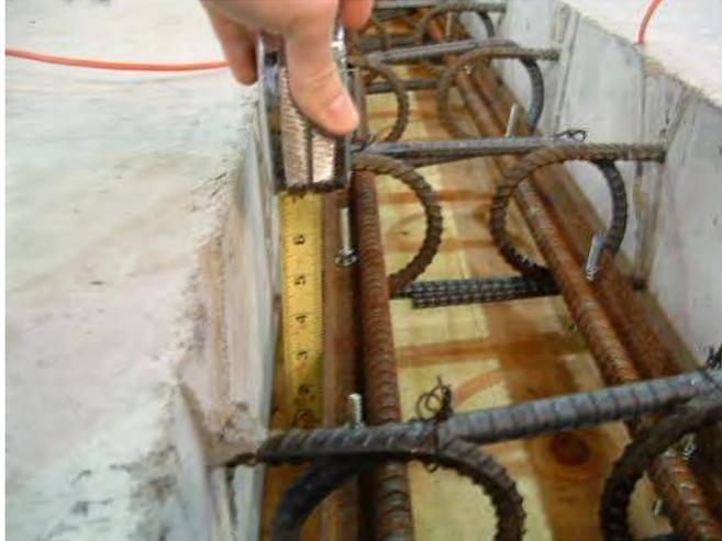
**Figure 31. Looped Reinforcing Bar Tied to Bars Extending From Panel**
