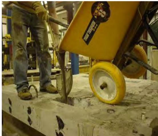
**Figure 34. Filling the Shear Pockets and Haunches With Grout**
