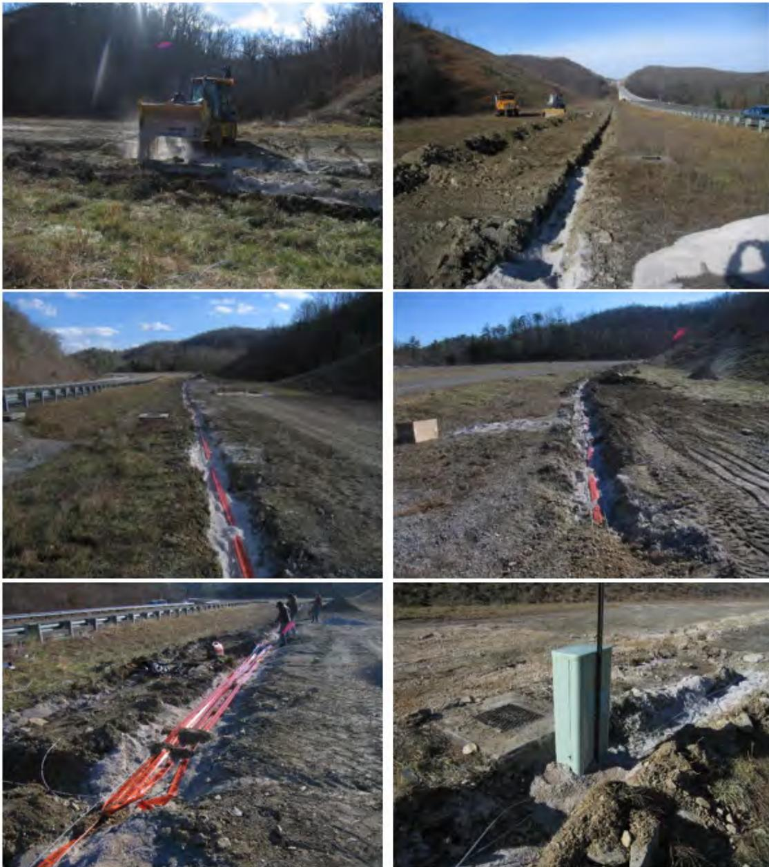
**Figure 4. Buried Cable Installation.** Trench being filled with fine aggregate (*top left*) and trench bedding after material was leveled (*top right*); cable placement on top of bedding material (*middle left*) and trench backfilling (*middle right*); lead-in cables overlapping along the detection line (*bottom left*) and processor enclosure location (*bottom right*).
