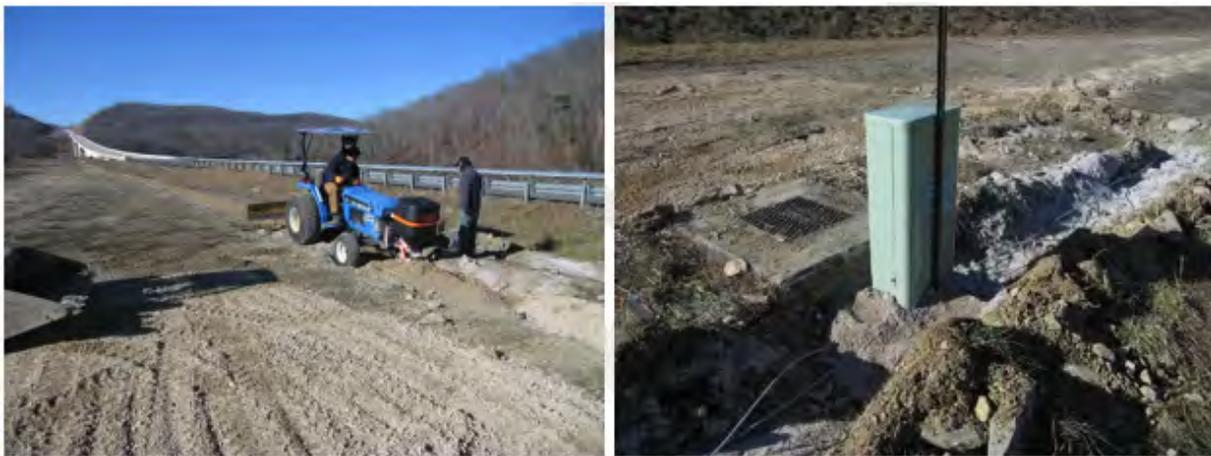
**Figure 5. Backfill Material Leveling (left) and Lead-in Cables Connected to the Processor Telecom Enclosure (right). The concrete utility vault can be seen in front of the enclosure.**
