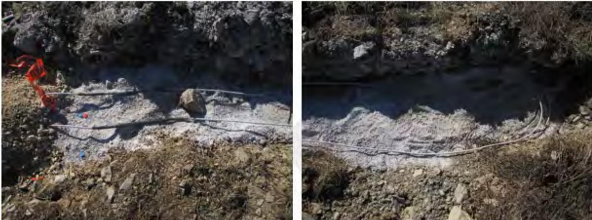
**Figure 6. Cable Ends Showing Decouplers (*left*) and Long Terminators (*right*) for Data Flow Termination**
