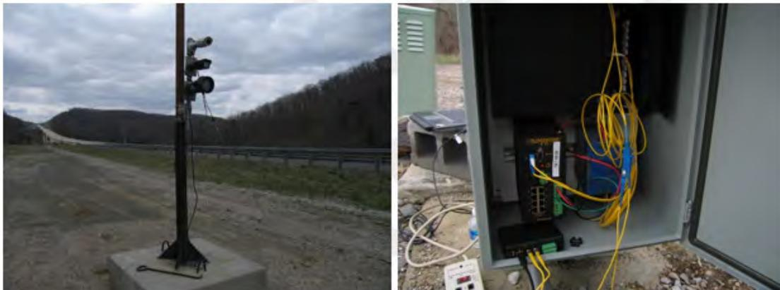
**Figure 13. Surveillance Camera (top) and Illuminators Used for Cable Monitoring (left) and Fiber Optic Connection to Smart Road Network (right). The NIU at the bottom was being tested to verify the connectivity and cable response to crossings.**
