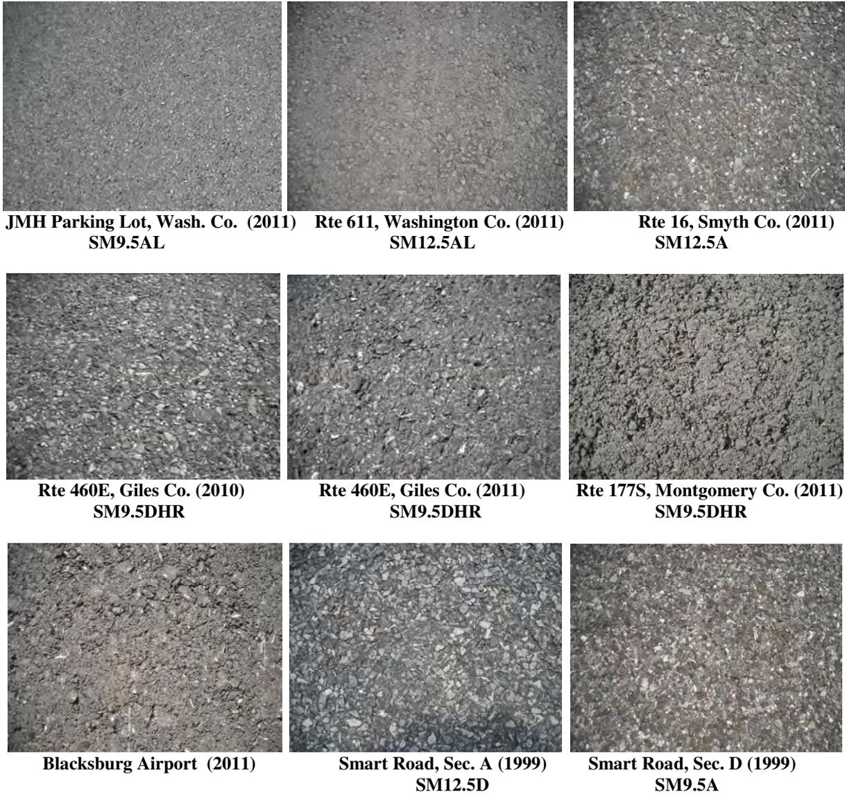
**Figure 7. Pavement Sections Selected for Friction/Texture Testing: Salem District. Images taken in 2012, placement year in parentheses.**
