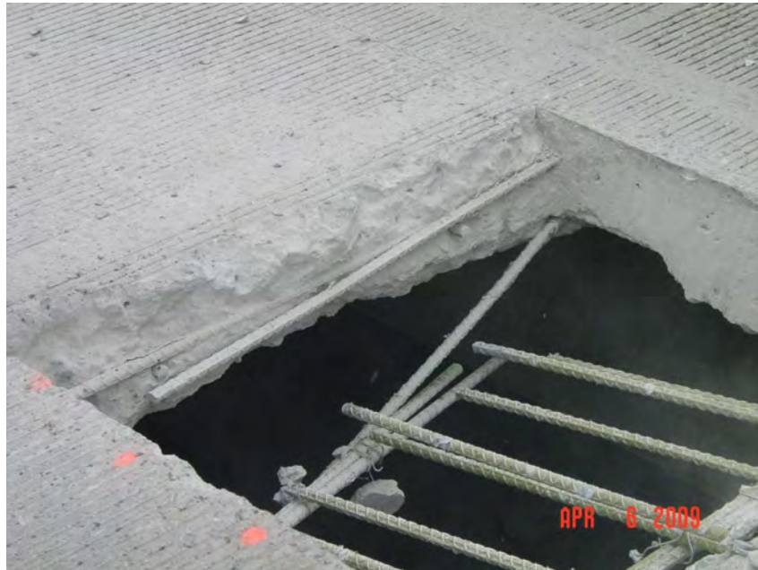
Figure 2. Failed Section of Closure Pour
