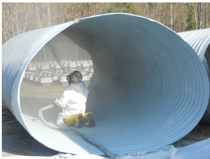
Figure 3. Installation of Spray-on Polyurea Liner
