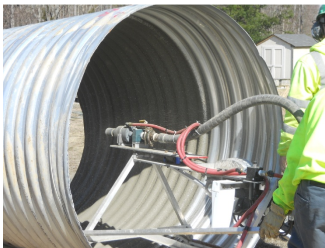
Figure 2. Installation of Cementitious Spray-on Liner
