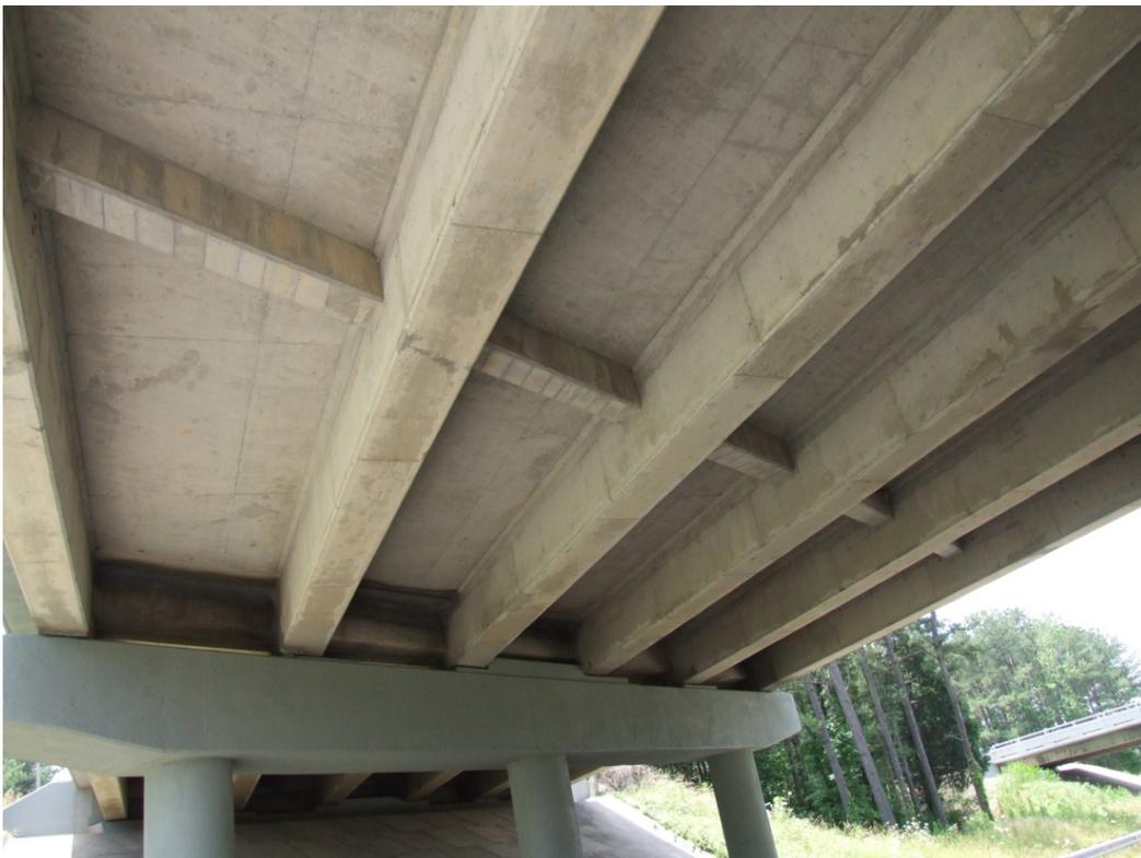
**Figure 6. Underside of Deck of I-85 Bridge NBL (looking south). Underside is in good condition and relatively free of leaking cracks. No full-depth patching was done.**
