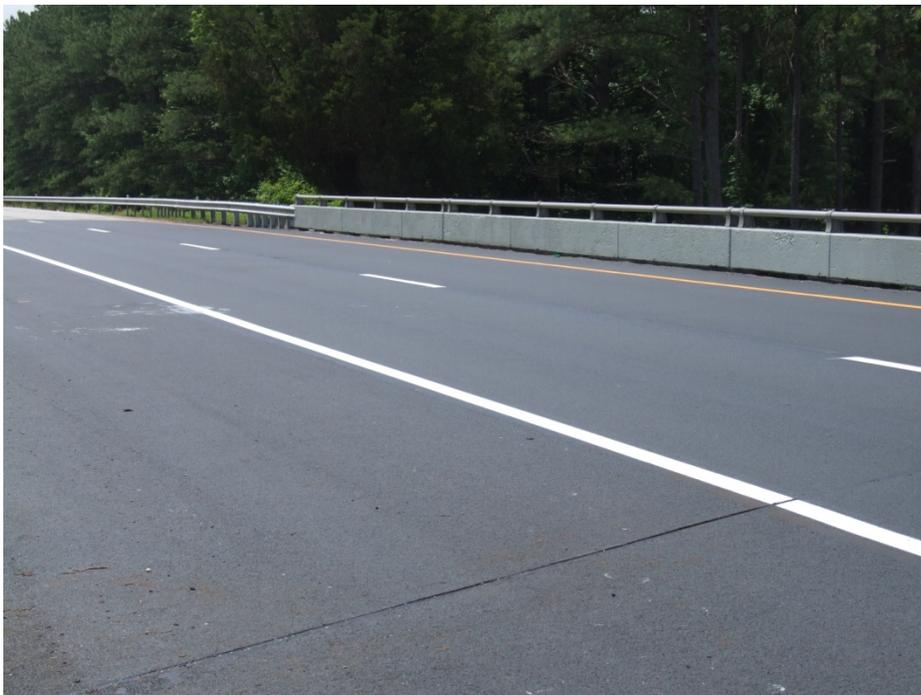
**Figure 2. Rosphalt Overlay on I-85 Bridge NBL (looking south). Lanes have saw-cut and sealed joints in Rosphalt between abutment and approach slab.**
