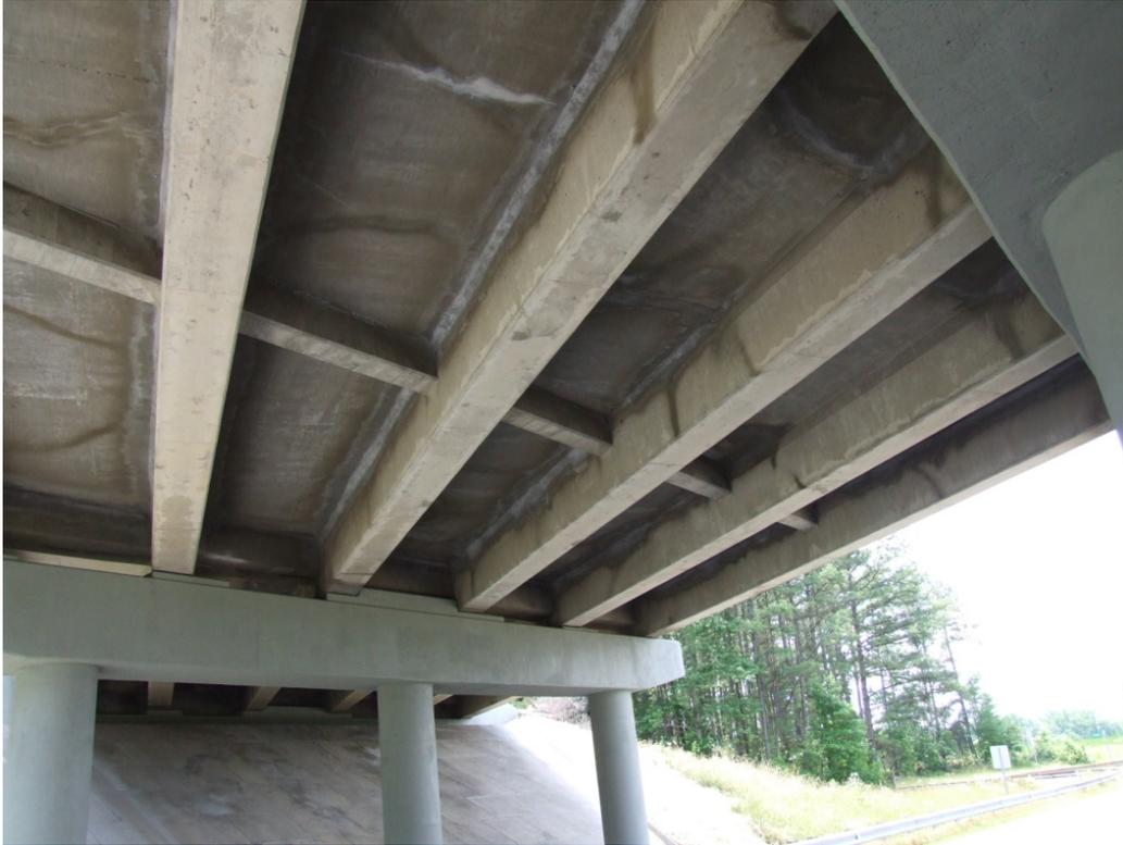
**Figure 5. Underside of Deck of I-85 Bridge SBL (looking south). Leaking cracks and many full-depth patches are shown.**
