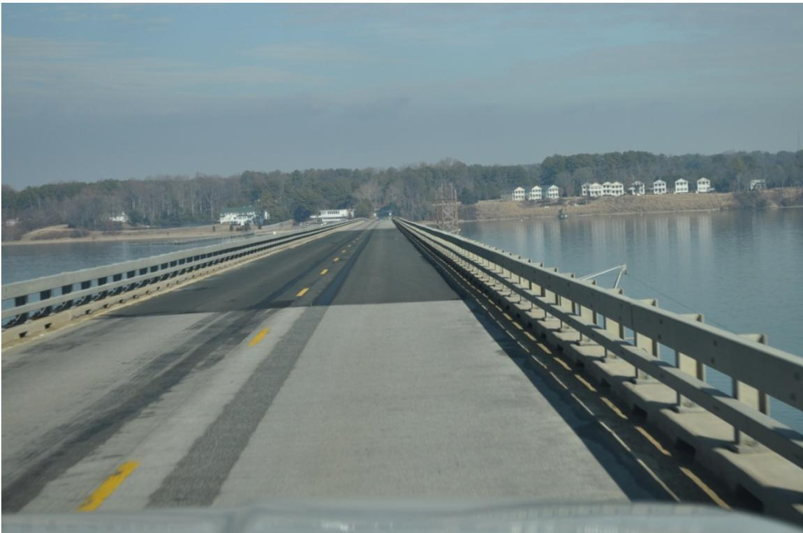
**FIGURE D1. Rosphalt Overlay on the Norris Bridge going eastbound toward White Stone**
