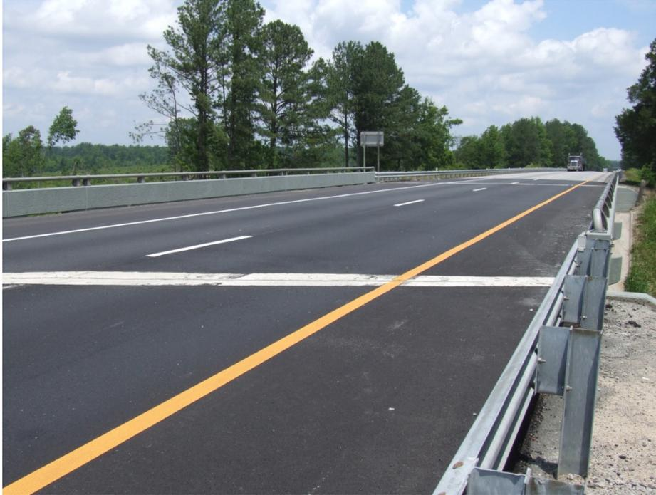
**Figure 1. SM-9.5 Asphalt Overlay on I-85 Bridge SBL (looking north). Lanes have sealed joints between concrete headers located above abutment and approach slab.**
