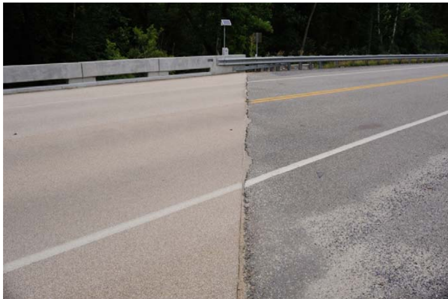
Figure 25. Approach at Abutment B (August 2011)
