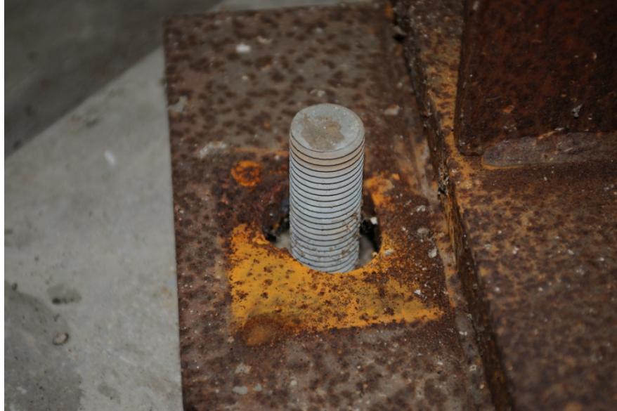
Figure 21. Sole Plate After Remedial Work
