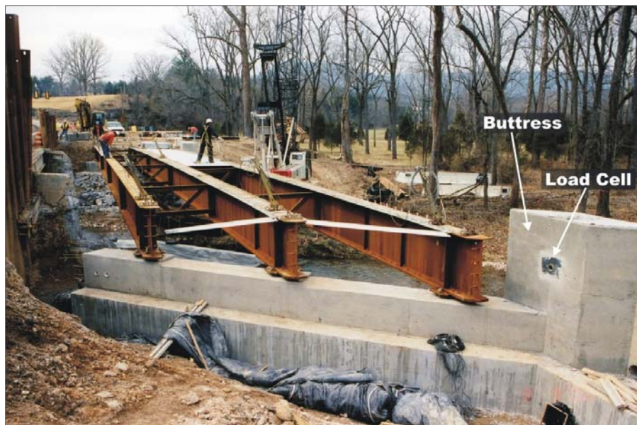
Figure 14. Buttress with Load Cell at Abutment B
