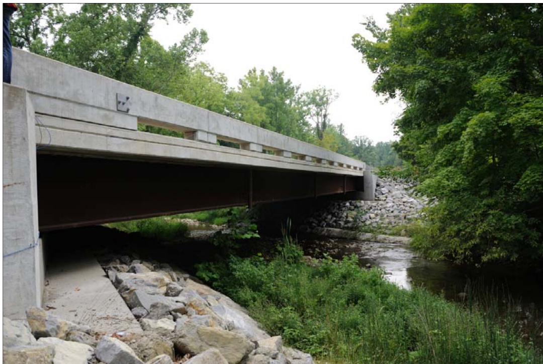
Figure 2. Semi-integral Bridge on Route 18 Over Blue Spring Run
