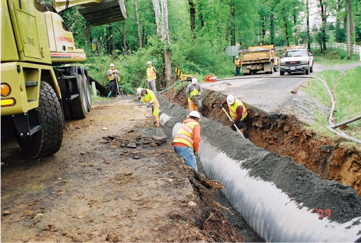
Figure 3. Installation of 48-inch Pipe at Route 684
