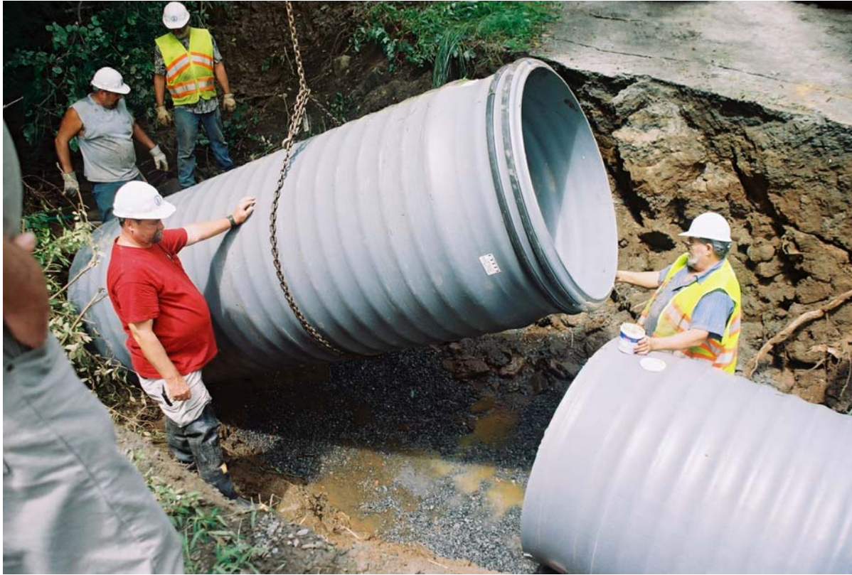
Figure 7. Installation of 48-inch Pipe at Route 698
