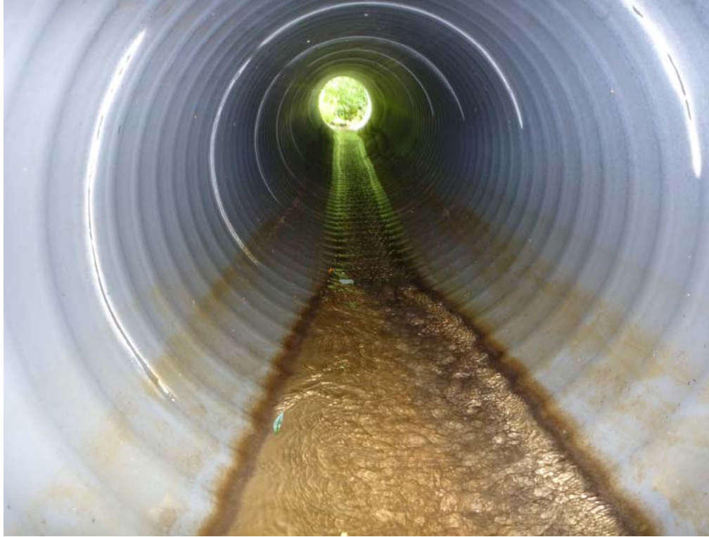
Figure 10. View of 30-inch Pipe at Route 635 After 1 Year in Service
