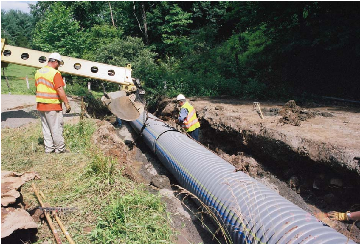
Figure 4. Installation of 30-inch Pipe at Route 736
