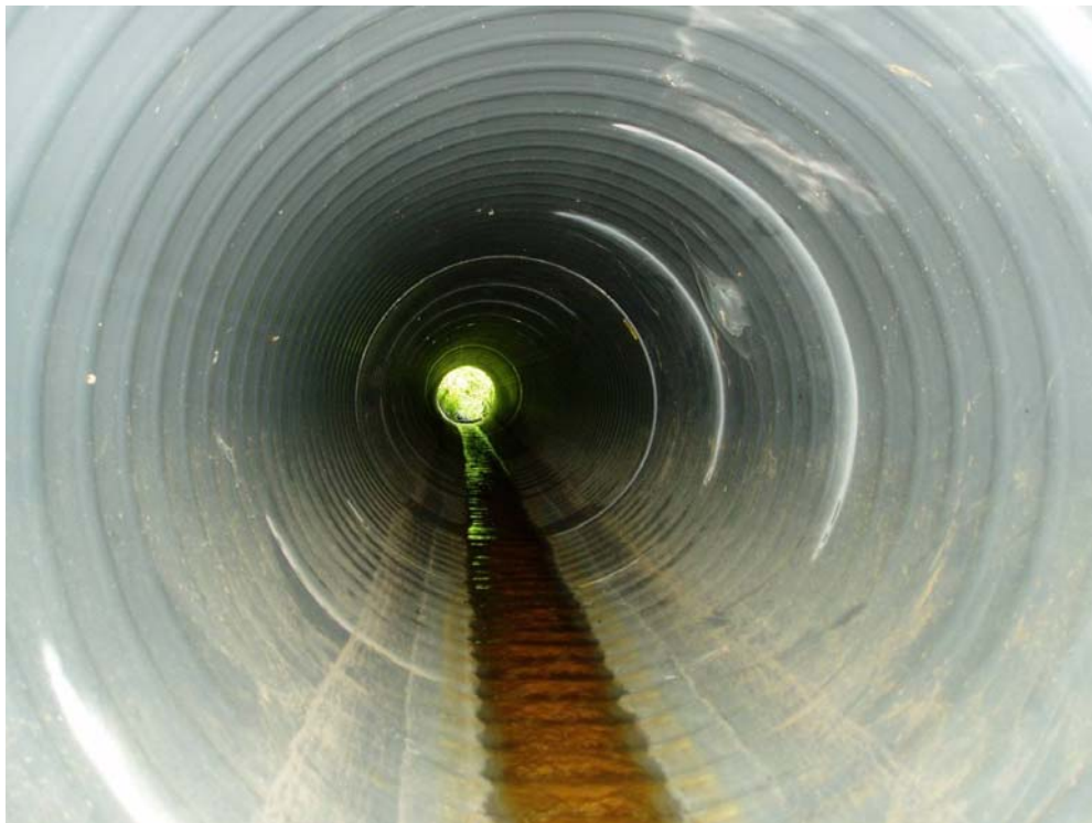
Figure 9. View of 30-inch Pipe at Route 736 After 1 Year in Service
