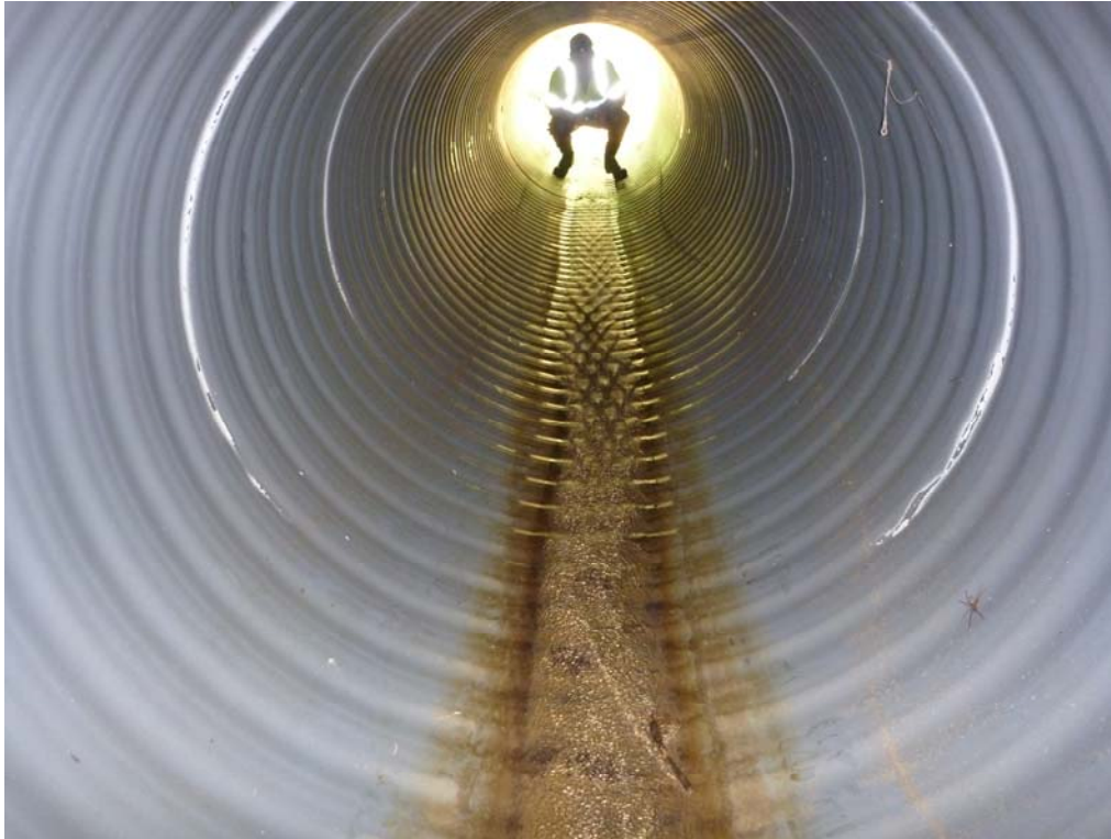
Figure 11. View of 48-inch Pipe at Route 635 After 1 Year in Service
