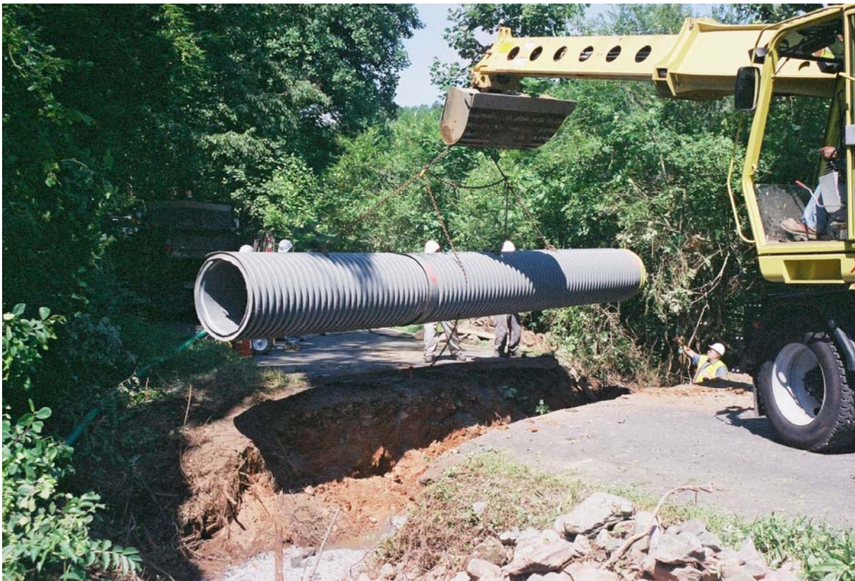
Figure 5. Installation of 30-inch Pipe at Route 635
