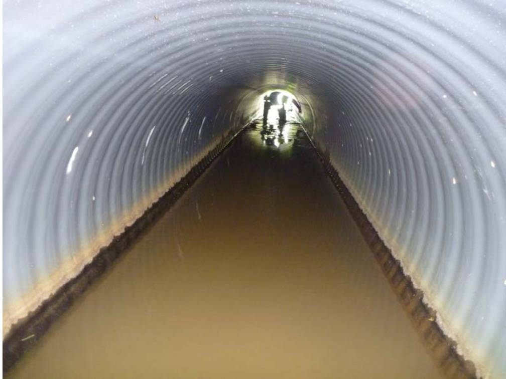
Figure 8. View of 48-inch Pipe at Route 684 After 1 Year in Service
