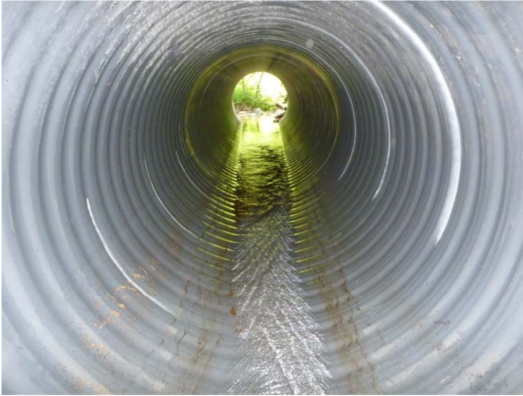
Figure 12. View of 48-inch Pipe at Route 698 After 1 Year in Service
