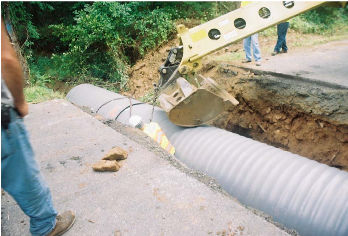
Figure 6. Installation of 48-inch Pipe at Route 635
