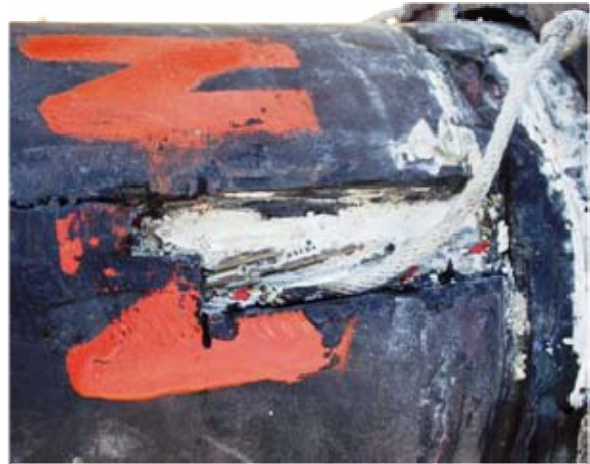
Figure 29. Top Left, Stay-cable prior to inspection; Top Right, Rubber boot removed and inspection location determined; Middle Left, Middle Right, and Bottom Left, Plastic removed to create portal for viewing; Bottom Right, Viewing portal opened and wires revealed for inspection.
