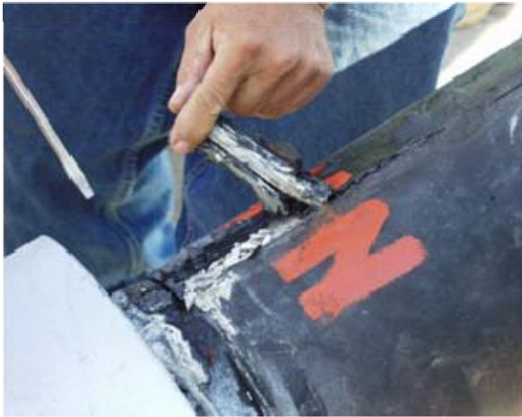
Figure 29. Top Left, Stay-cable prior to inspection; Top Right, Rubber boot removed and inspection location determined; Middle Left, Middle Right, and Bottom Left, Plastic removed to create portal for viewing; Bottom Right, Viewing portal opened and wires revealed for inspection.
