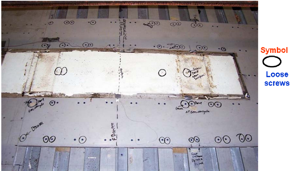
Figure 17. Loose screws
