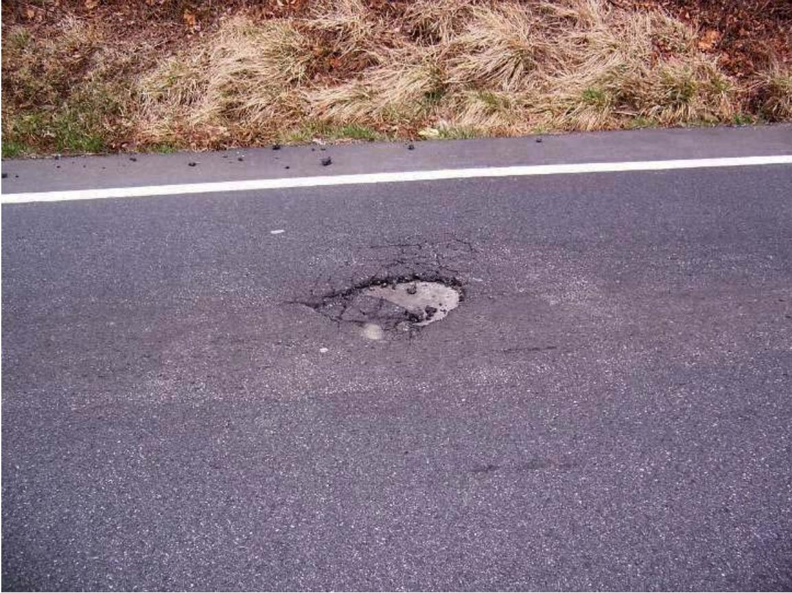
**Figure 1. Delamination Pothole**
