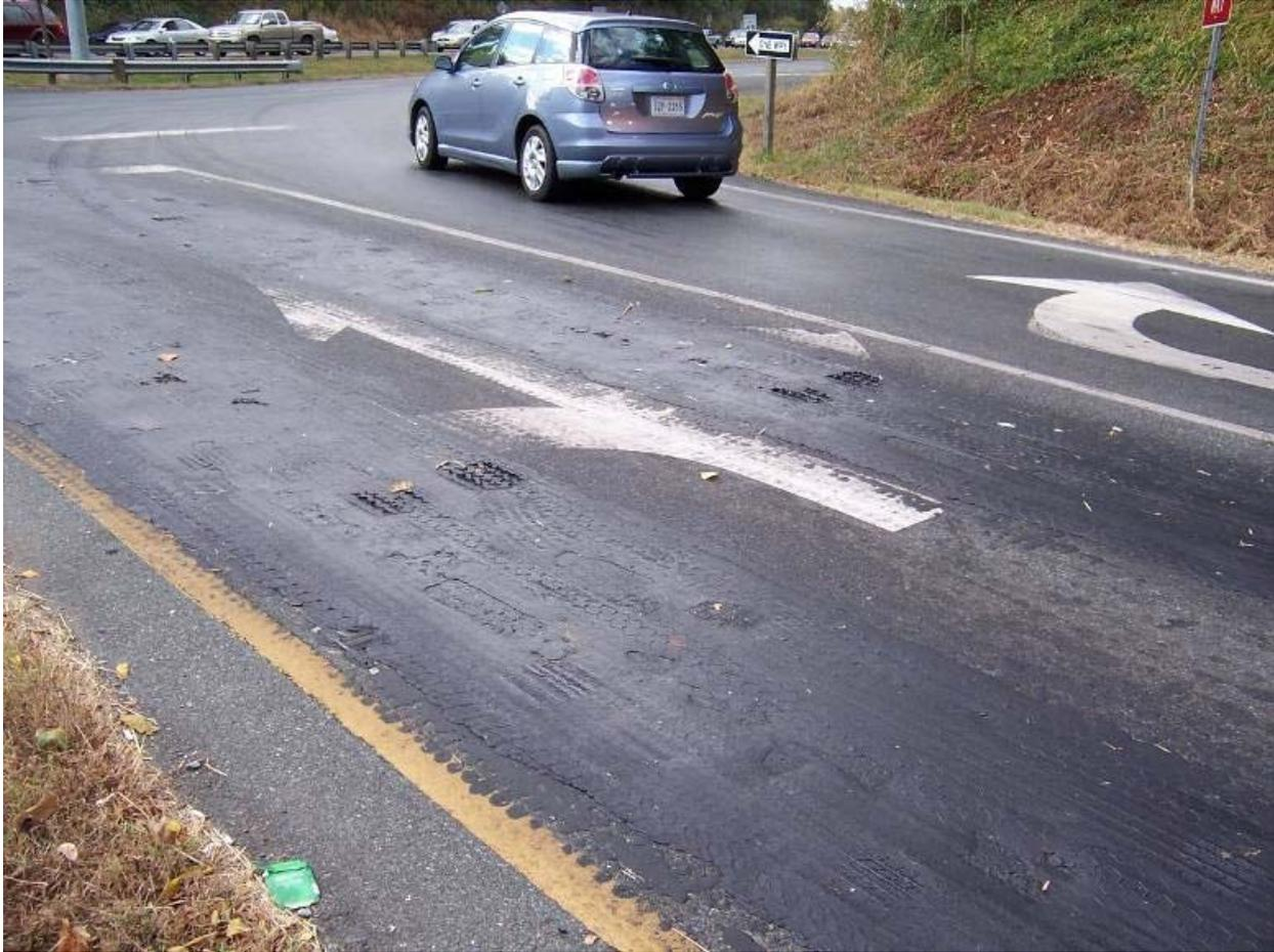
**Figure 2. Tack Build-up at Intersection.**
