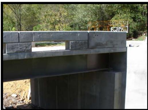
Figure 22. Guardrail Attachment Absent
