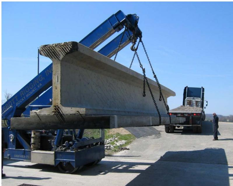
**Figure 24. Removal of one half of the PCBT-53**
