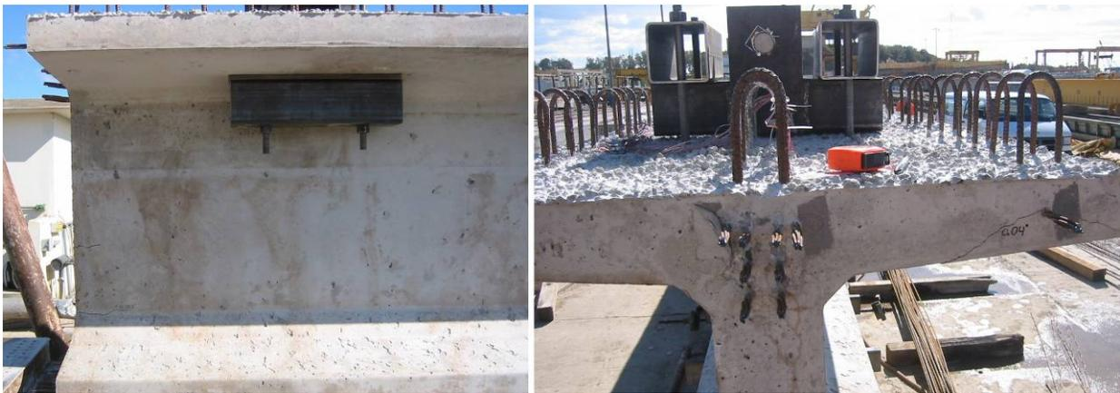
**Figure 7. Girder lifting device**
