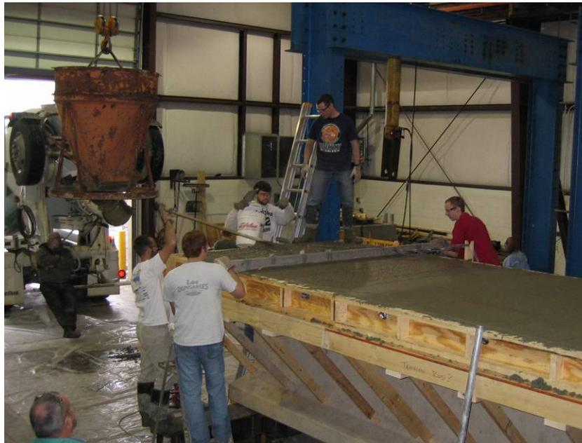
**Figure 11. Deck concrete placement**
