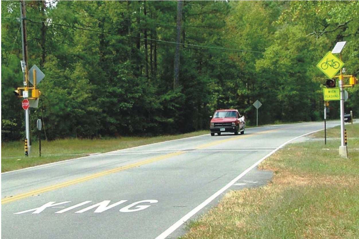
Figure 1. Cross Alert System on Route 5 in James City County, Virginia. The photograph was taken prior to the official opening of the Chickahominy Riverfront Phase on May 1, 2007.
