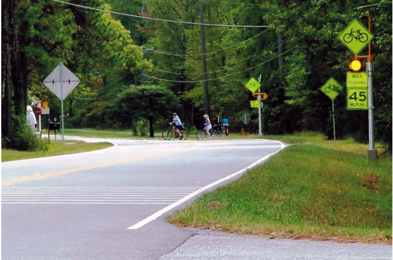
Figure B3. Route 5 Eastbound Approach to Crossing
