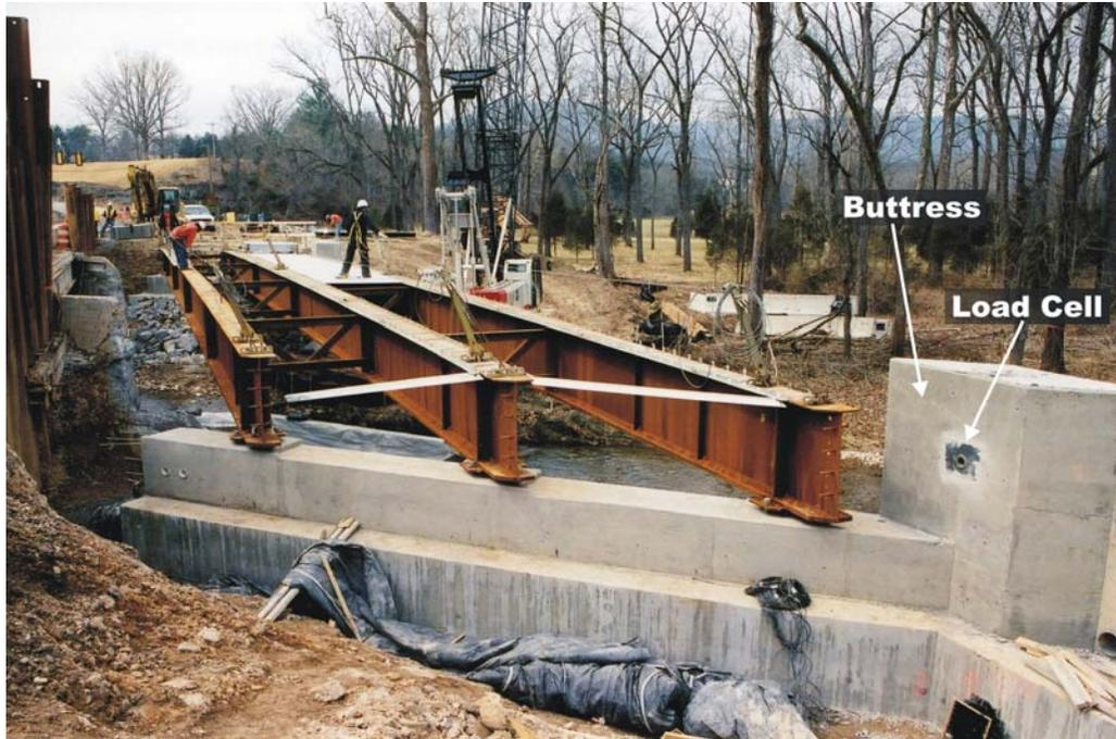
**Figure 6. Concrete Buttress at Abutment B**
