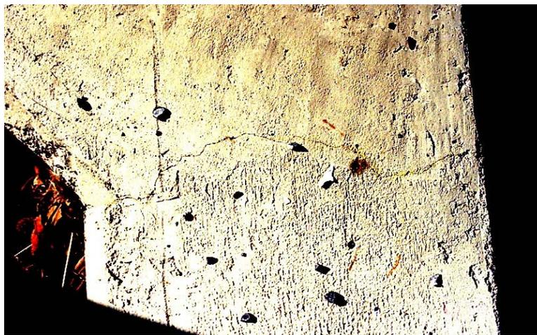
**Figure 19. Plan View of Cracked Wingwall at Abutment B**
