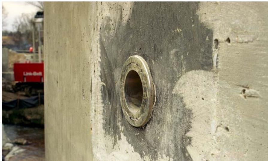
**Figure 7. Load Cell at Buttress of Abutment B**
