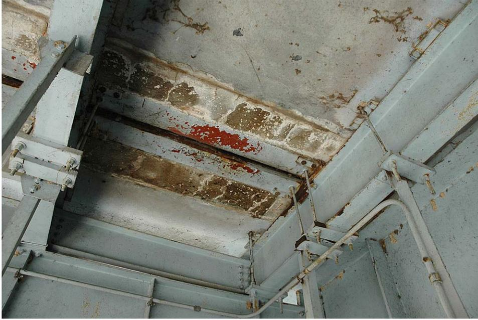
**Figure 12. More Efflorescence and Rust Staining at Closure Pours**
