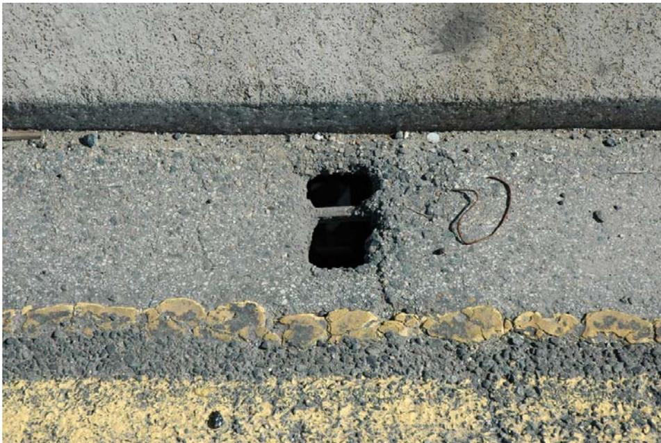
**Figure 7. Drainage Scupper Partially Obstructed by Asphalt Overlay**
