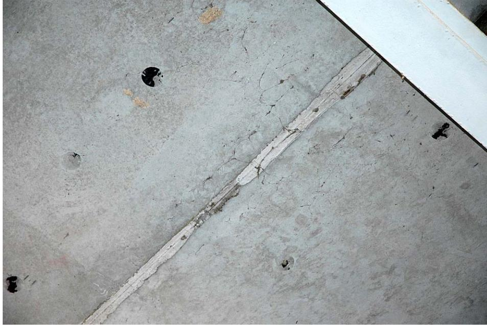
**Figure 10. Underside of Adjacent Deck Panels and Accompanying Joint in Good Condition**
