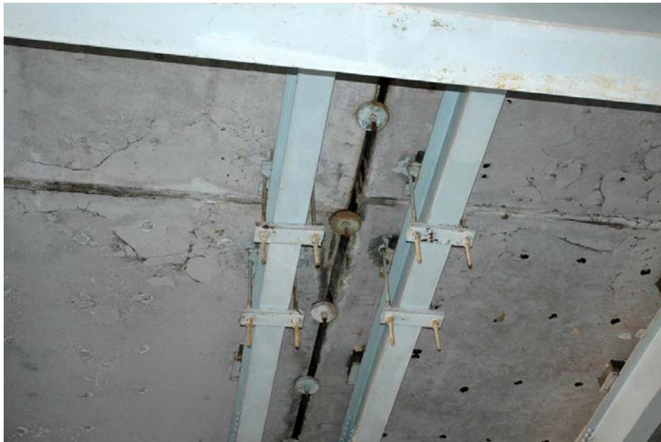
**Figure 9. Median Barrier Connection to Underside of Full-Depth, Precast Concrete Deck Panels. The black circles are plastic reinforcing bar chairs used during the fabrication process.**
