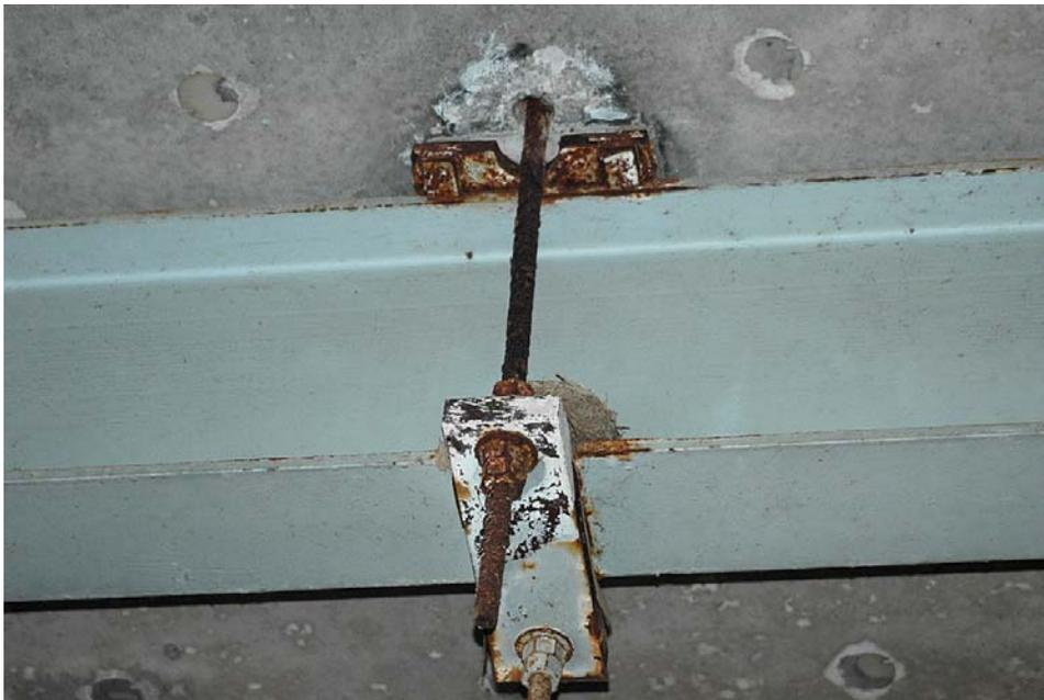
**Figure 15. Corroded Hold-Down Bar Connecting Deck to Stringer**
