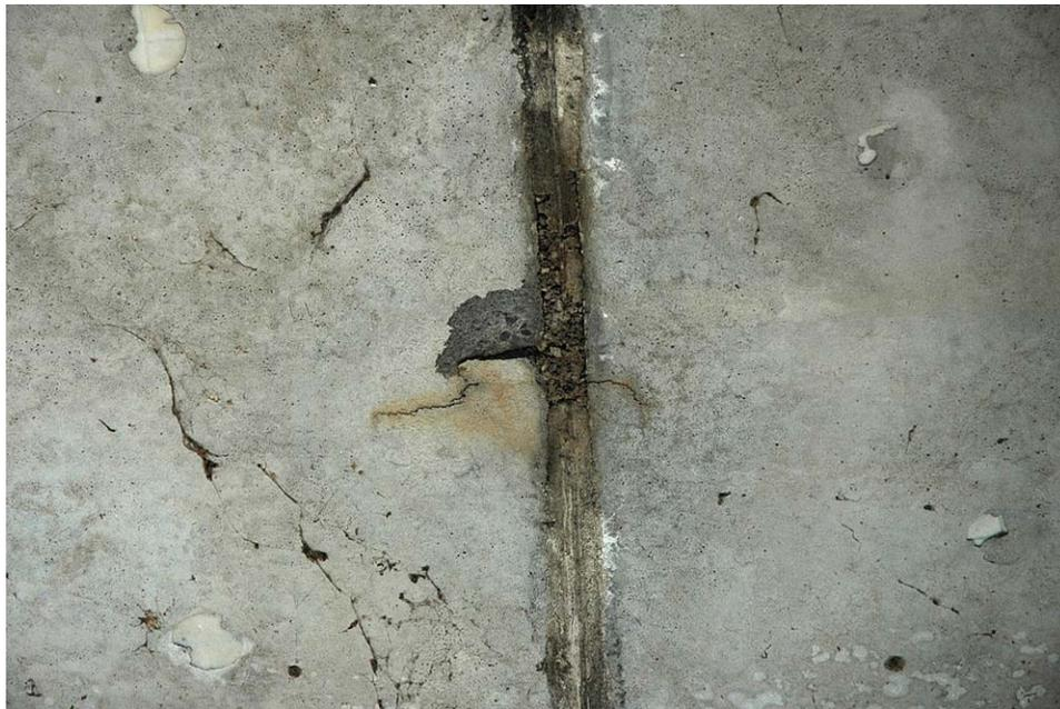
**Figure 11. Panel Joint with Rust Staining and Spall**
