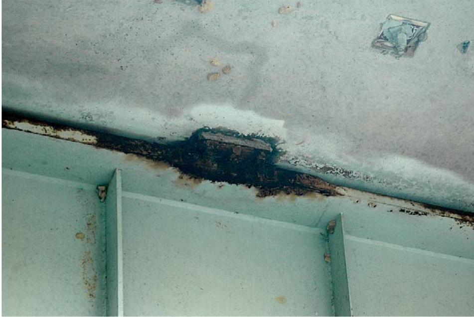
**Figure 14. Bearing Seat Subject to Corrosion**
