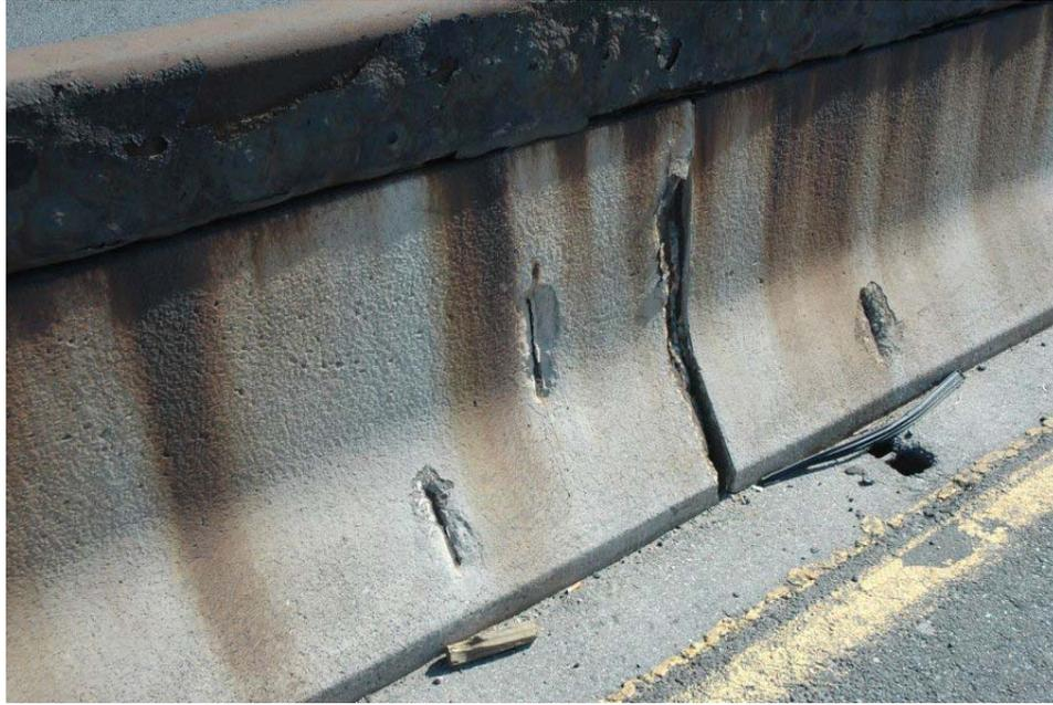
**Figure 8. Concrete Spalls Attributable to Rusted Rebar in Median Barrier**
