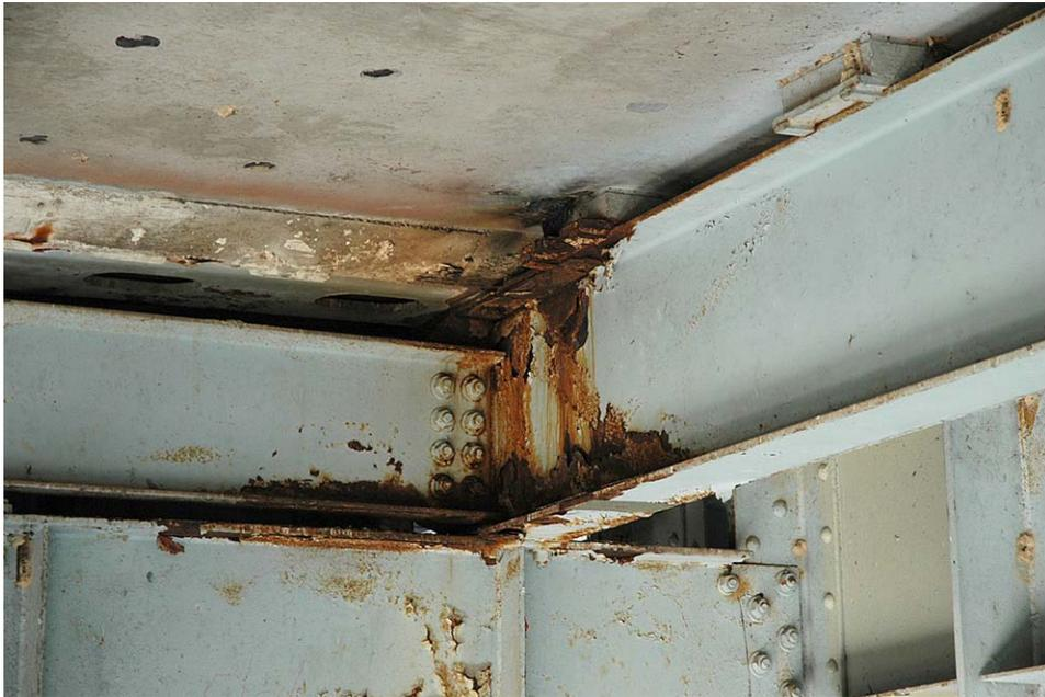
**Figure 13. Corroded Steel at Expansion Joint**
