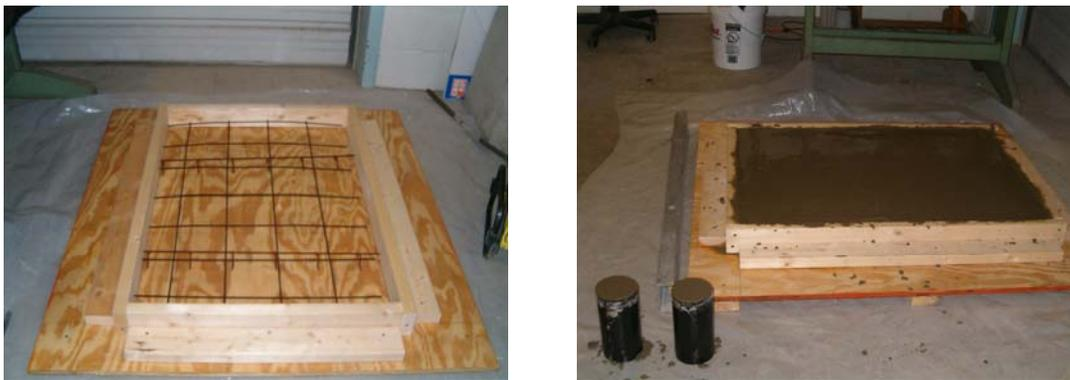
**Figure 18. Plywood form created with reinforcing steel, and concrete slab poured**
