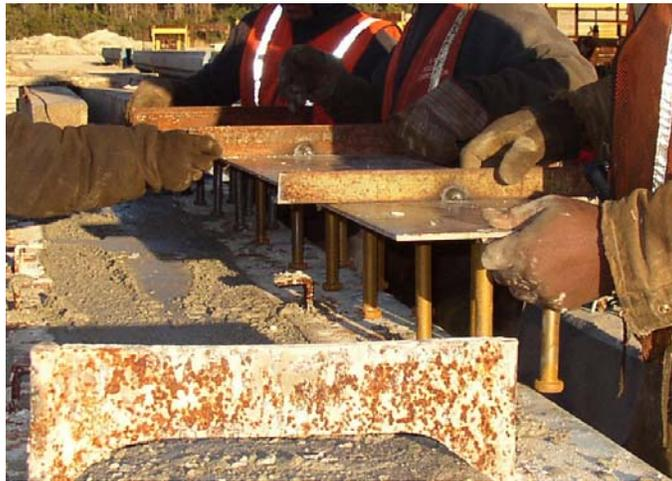
**Figure 2. New Detail For Horizontal Shear Reinforcement**
