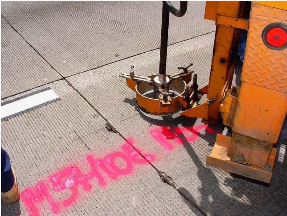
**Figure 12. Field Coring Operation Near Joint 54 on I-66**
