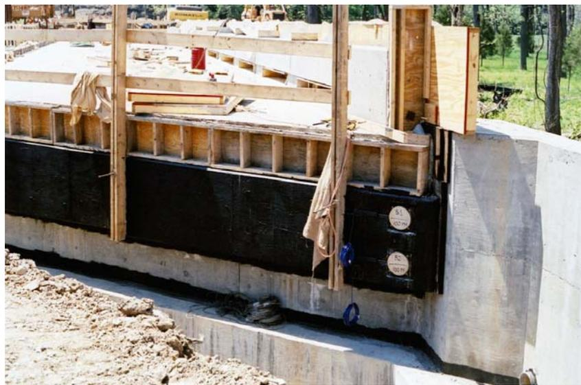
**Figure 13. Earth Pressure Cells at Abutment B**
