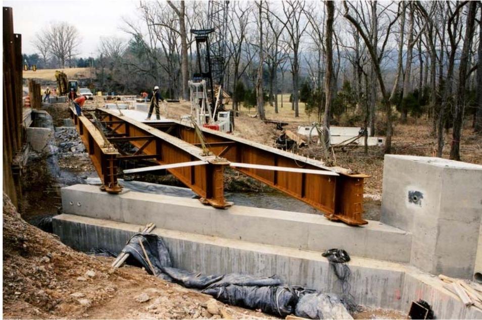
**Figure 6. Placement of Structural Steel**
