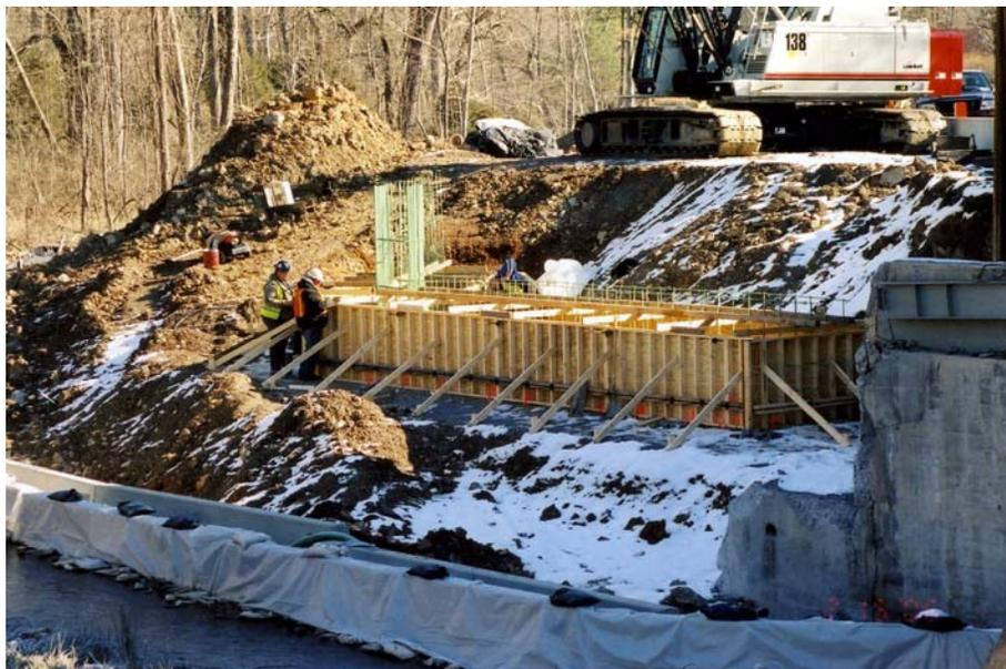
**Figure 5. Formwork for Abutment B**
