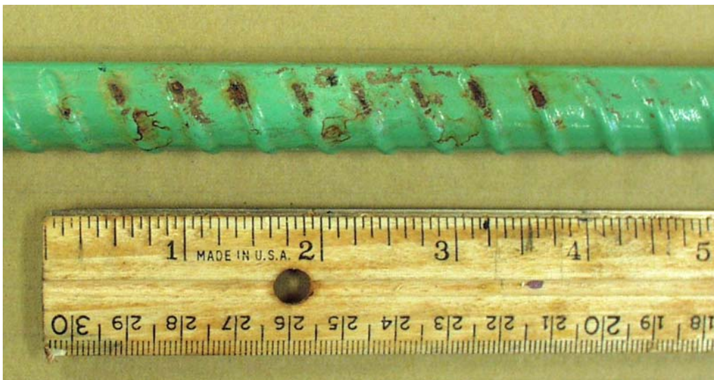
Figure 6. Damaged Region Along Epoxy-Coated Rebar
