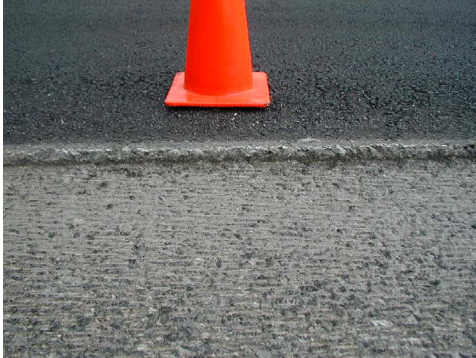
Figure 6. Micro-milled Surface
