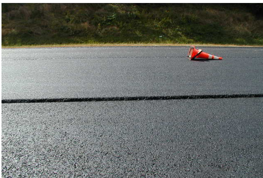
Figure 8. Drop-off Edge for Straight Overlay Operation
