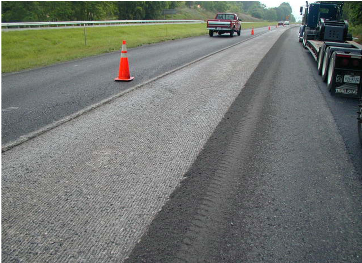
Figure 5. Micro-milled Surface
