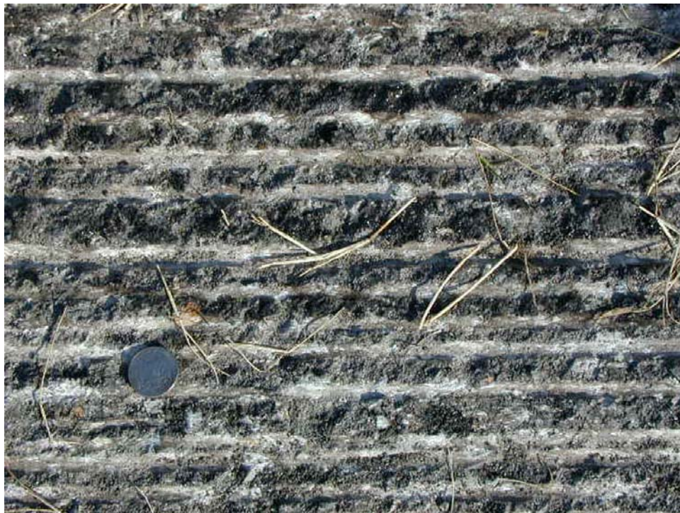
Figure 7. Conventional-Milled Surface
