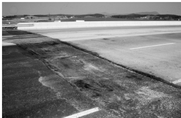
Figure 16. Roadway Approach at the Route 257 Integral Backwall Bridge
