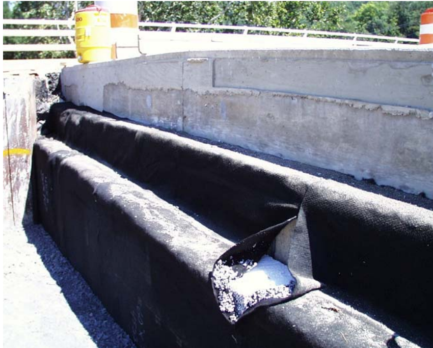
Figure 4. Elasticized EPS at the Backwall
