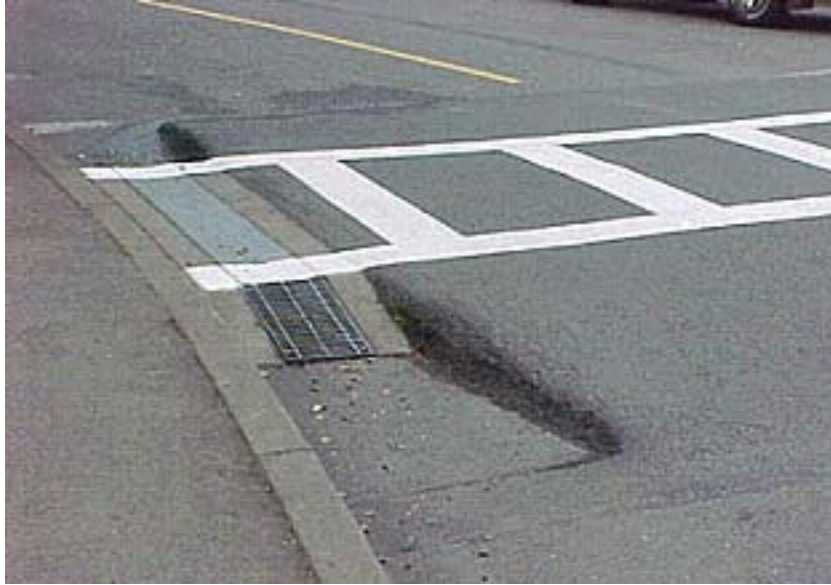
Figure B5. Raised Mid-block Crossing. From http://pedbikeimages.org/ / Portland Office of Transportation. Reprinted with permission.
