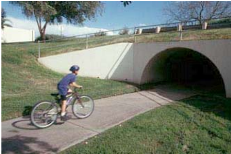
Figure B19. Grade-Separated Crossing (Tunnel) Under a Roadway. From www.pedbikeimages.org/ Dan Burden. Reprinted with permission.
