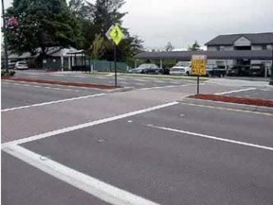
Figure B6. Example of a Textured Pavement Crosswalk. From www.pedbikeimages.org / Dan Burden. Reprinted with permission.
