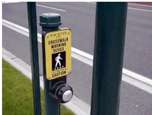
Figure B15. Pedestrian Pushbutton for Flashing Beacon Operation. From www.pedbikeimages.org/ Dan Burden. Reprinted with permission.
