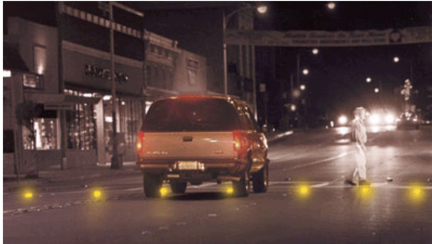
Figure B16. In-Roadway Warning Lights at a Mid-block Crosswalk. From www.pedbikeimages.org / ITE Pedestrian Bicycle Council. Reprinted with permission.
