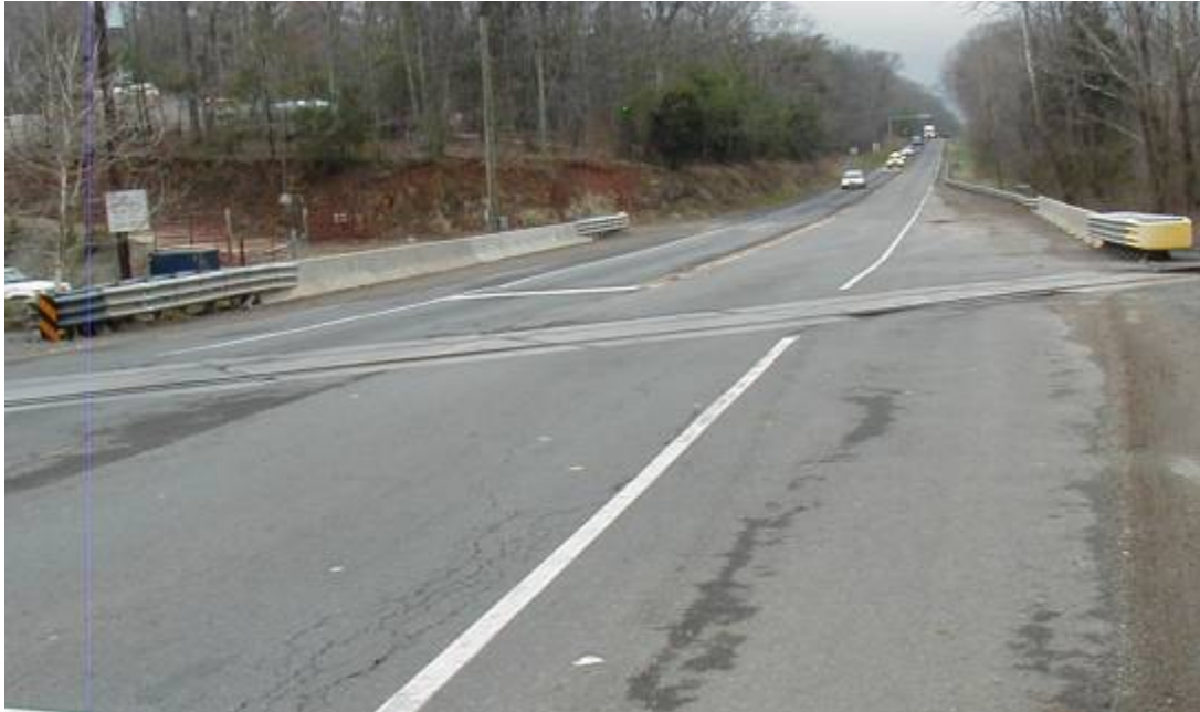
Figure 3. Overview of crossing at U.S. Route 15 (facing south).
