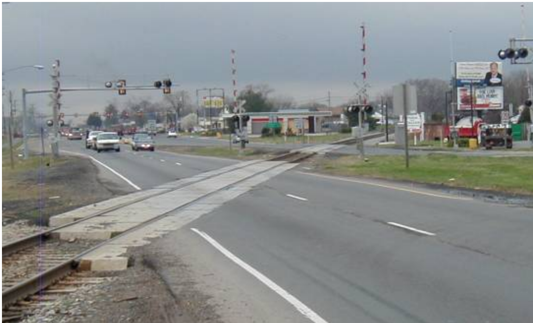
Figure 2. Overview of crossing at U.S. Route 29 (facing south).
