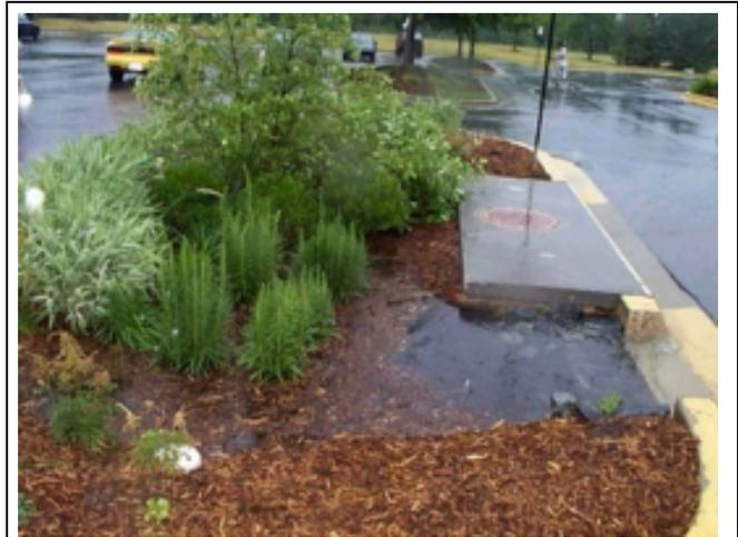
**Figure 5.2 - Typical “Rain Garden” Bioretention System**
