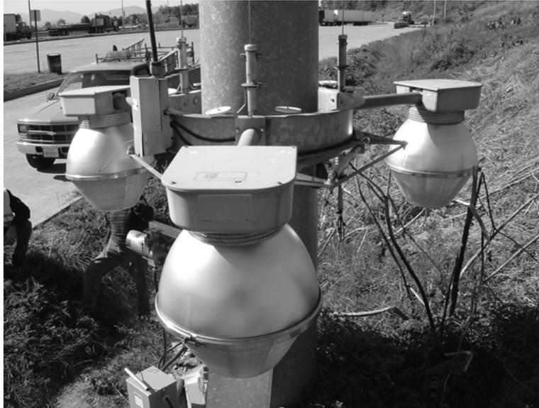
**Figure 6. HOLOPHANE® Lowering Device Ring/Light System at I-81 Troutville, Virginia Weigh Station**
