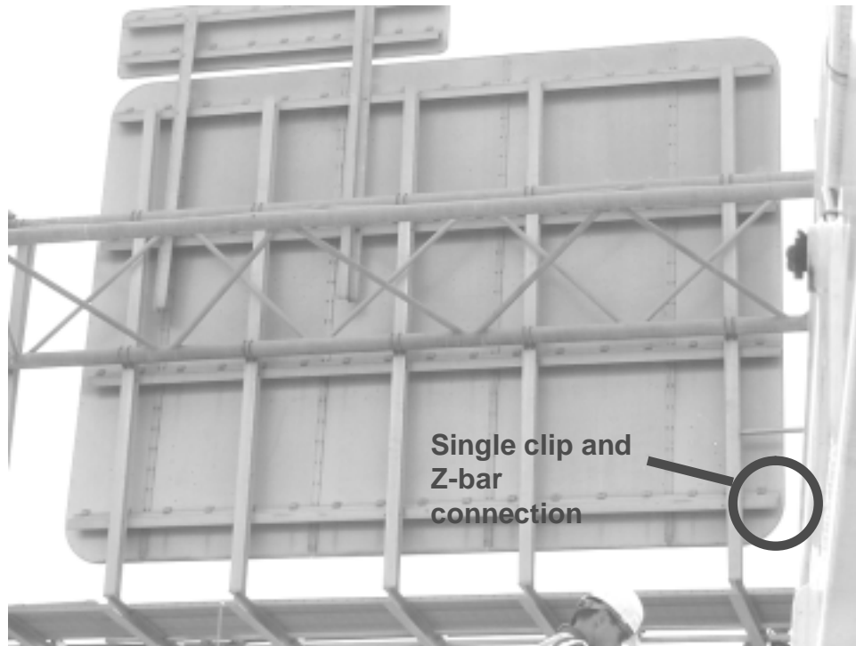
Figure 9. Sign Connected to Support.
