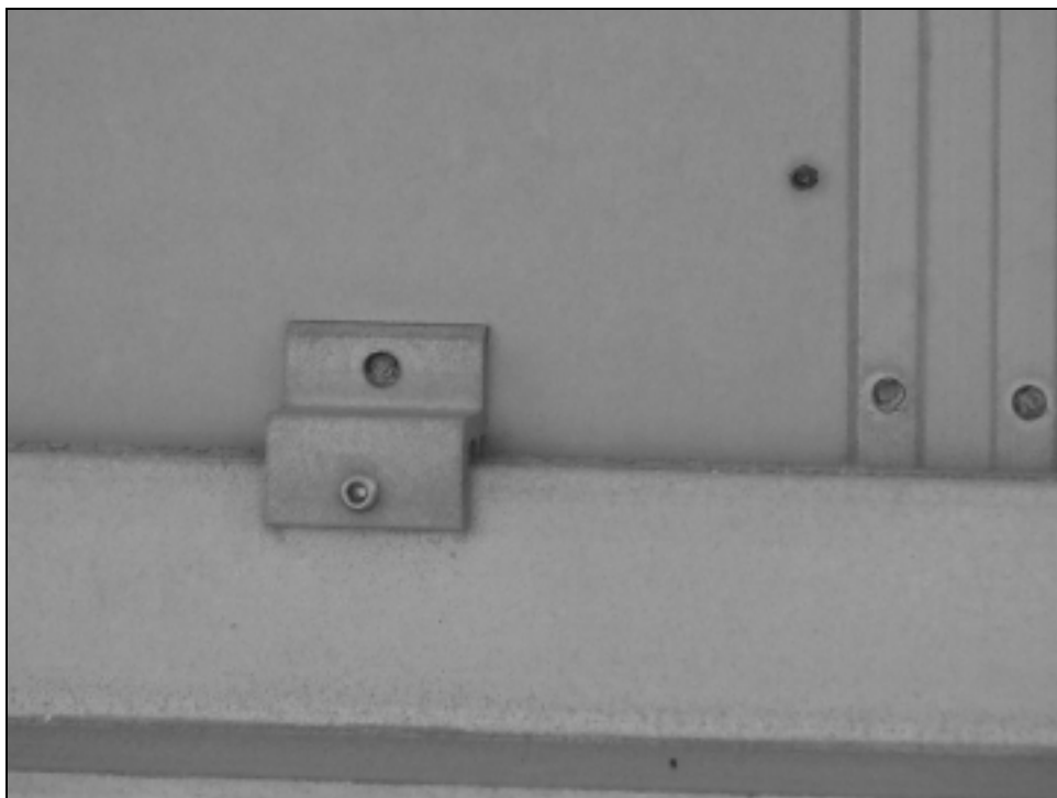
Figure 11. Failed Stud on Sign.
