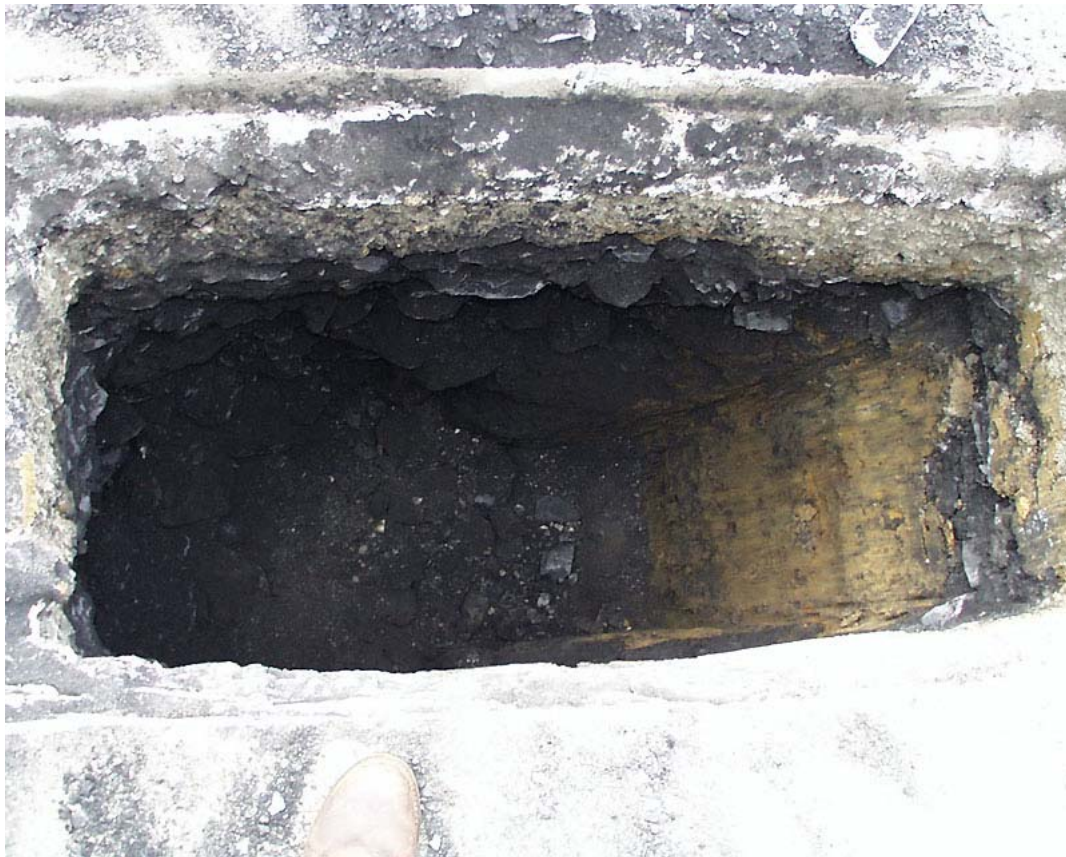
Figure 4. Test Pit Excavation of Culvert Trench.
