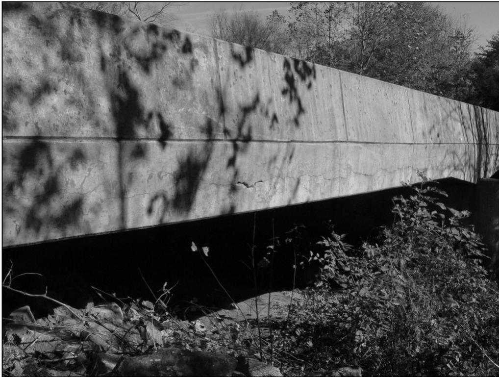
**Figure 4. Crack along length of bridge.**
