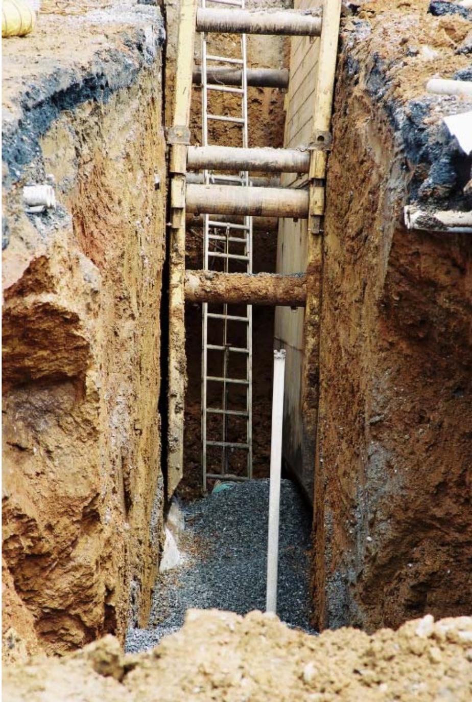
**Figure 6-5. Open Trench with Safety Box and Monitoring Well**
