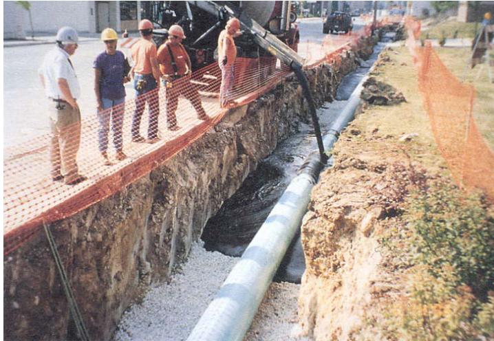
Figure 4-2. Placement of Flowable Fill (Ramme 1999)
