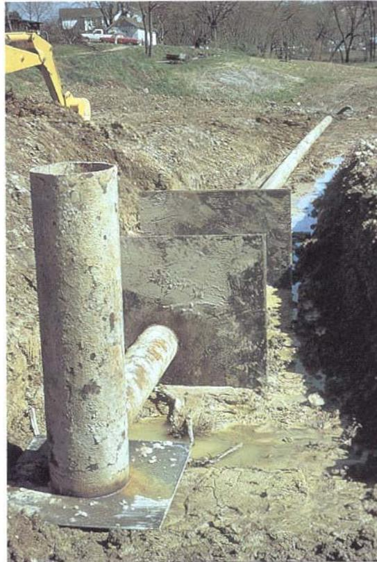
**Figure 4-5. Anti-seep Collar in a Pond Embankment**
