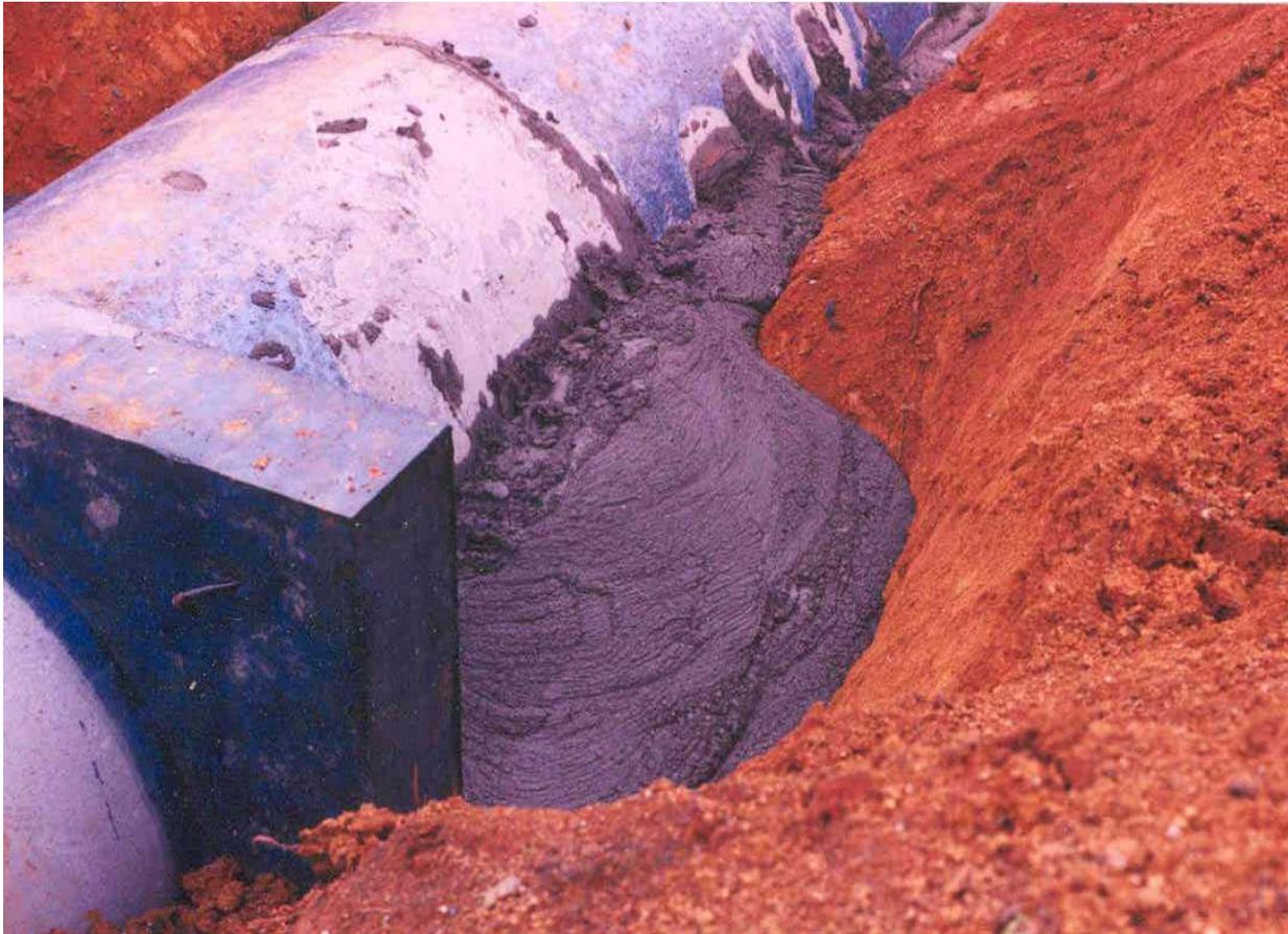
**Figure 6-16. Flowable Backfill installed around bottom portion of pipe (Davis 2002A).**
