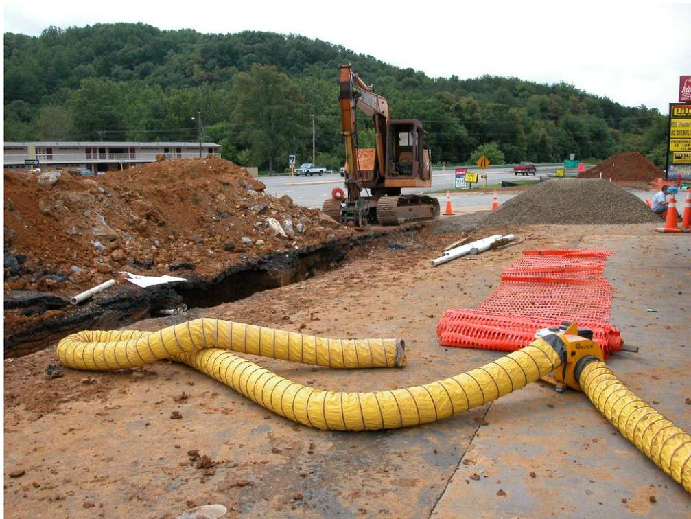
**Figure 6-8. Vapor Extraction Fan**
