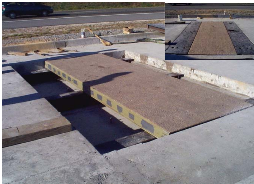
Figure 8 FRP deck field testing facility at the weight station
