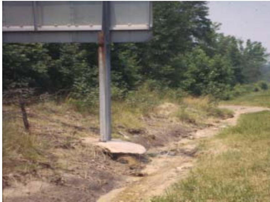
**Figure 4. Sulfide-bearing sediments of the Chesapeake Group are exposed along this stretch of I-95 in Spotsylvania County.** The stability of this signpost is compromised due to concrete degradation from acid attack. Furthermore, acid conditions (soil pH ~ 2.5) limit vegetative growth, which makes these sites particularly prone to erosion.
