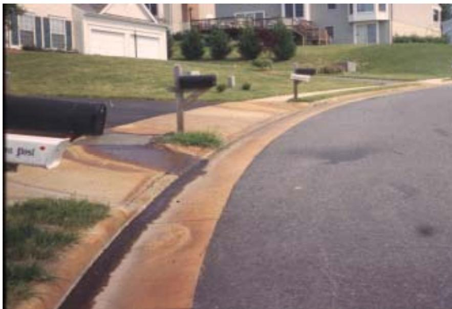
**Figure 5. Acid drainage from the Quantico slate in Stafford, Virginia, has caused extensive iron-staining along curbs and sidewalks through the Hampton Oaks subdivision.** Also, concrete etching occurs when acid drainage “dissolves” out the cement, deteriorating the concrete. Homeowners in this neighborhood apply the equivalent of 2 Mg agricultural lime per hectare per month to maintain soil pH above 5.5.
