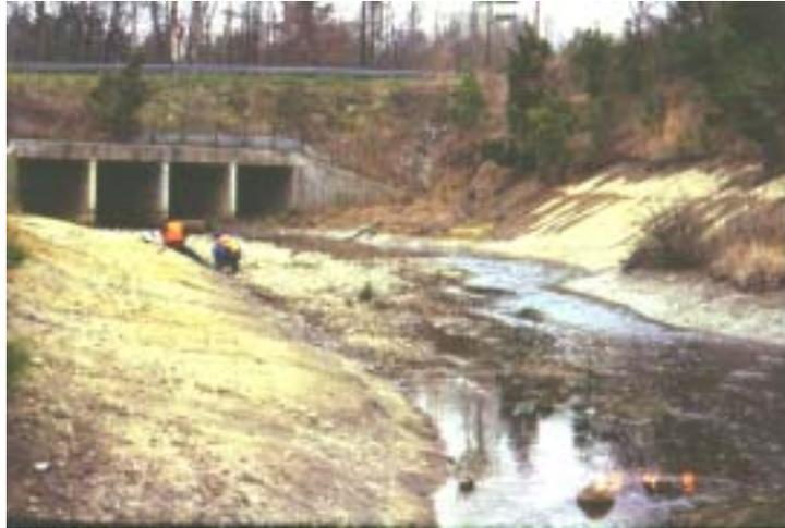
**Figure 6. Proctor's Creek was redirected due to road construction near the intersection of Rts-288 and 156 in Chesterfield County.** The creek was routed into an excavated channel through Lower Tertiary deposits. Extremely acid soil conditions ( $\text{pH} < 2.5$ ), which developed upon oxidation of the sediments, have inhibited vegetation along the stream bank.
