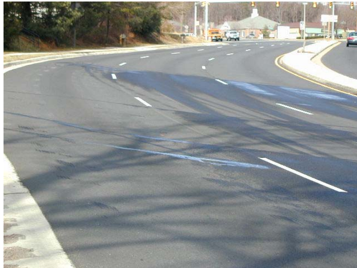
Figure 1. Drainage Across Old Bridge Road (After Coring)
