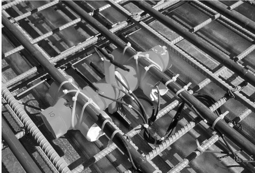
**Figure 7. View of Temperature Probe Module Attached to Heat Pipes**
