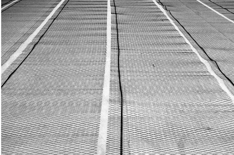
**Figure 7. Strips of Catalyzed Titanium Mesh Placed Over First Layer of Felt**
