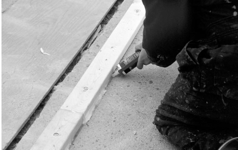
**Figure 5. Installation of Ponding Dam with Wood Strips and Silicone Caulk**
