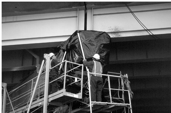
**Figure 11. Wrapping of Fiber-Encapsulated Pier Cap with Heavy Plastic Sheet to Keep Cellulose Fibers in Place and Wet During treatment**
