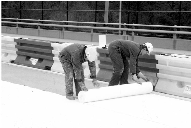
**Figure 6. Placement of First Layer of Felt Within Ponding Dam on Deck Span to Be Treated**
