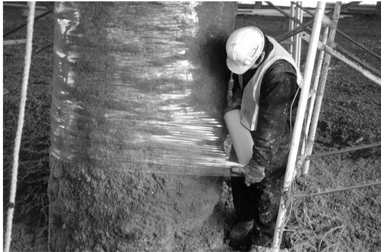
**Figure 12. Wrapping of Fiber-Encapsulated Pier Column, From Top to Bottom, with Self-Clinging Transparent Plastic Film**
