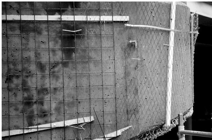
**Figure 9. Steel Mesh and Titanium Mesh Secured Over Straight Section and Curved End, Respectively, of Pier Cap**
