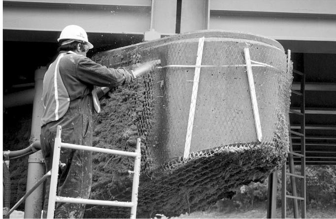
**Figure 10. Spraying of Wet Cellulose Fibers Over Pier Cap to Encapsulate Mesh Anode and Cap**
