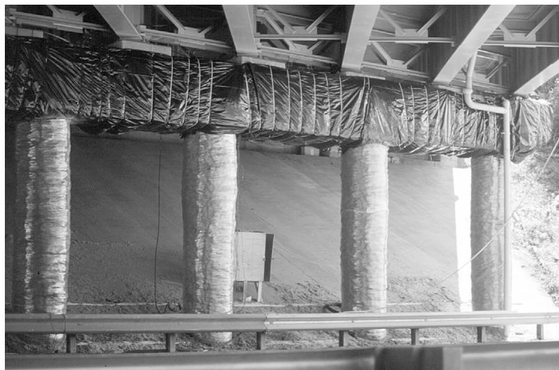
**Figure 13. Pier After Installation of Anode System.** Notice the wooden box where one of the rectifiers was housed during treatment.
